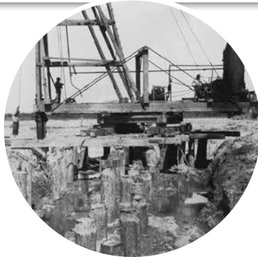
Construction begins on the Bonnet Carré Spillway.
