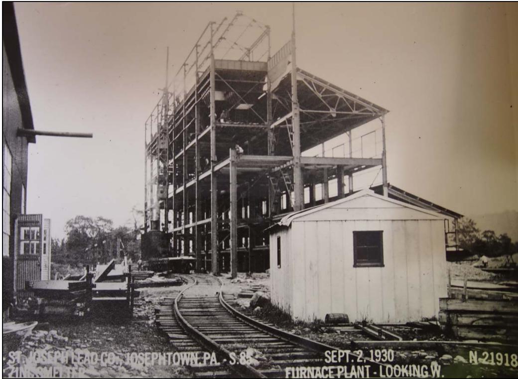
Figure 7. Furnace plant construction, September 2, 1930.
