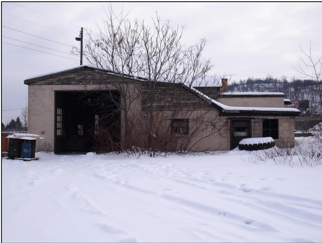
Photo 45. Garage (SC-32), front (north) façade and west elevation, view southeast
