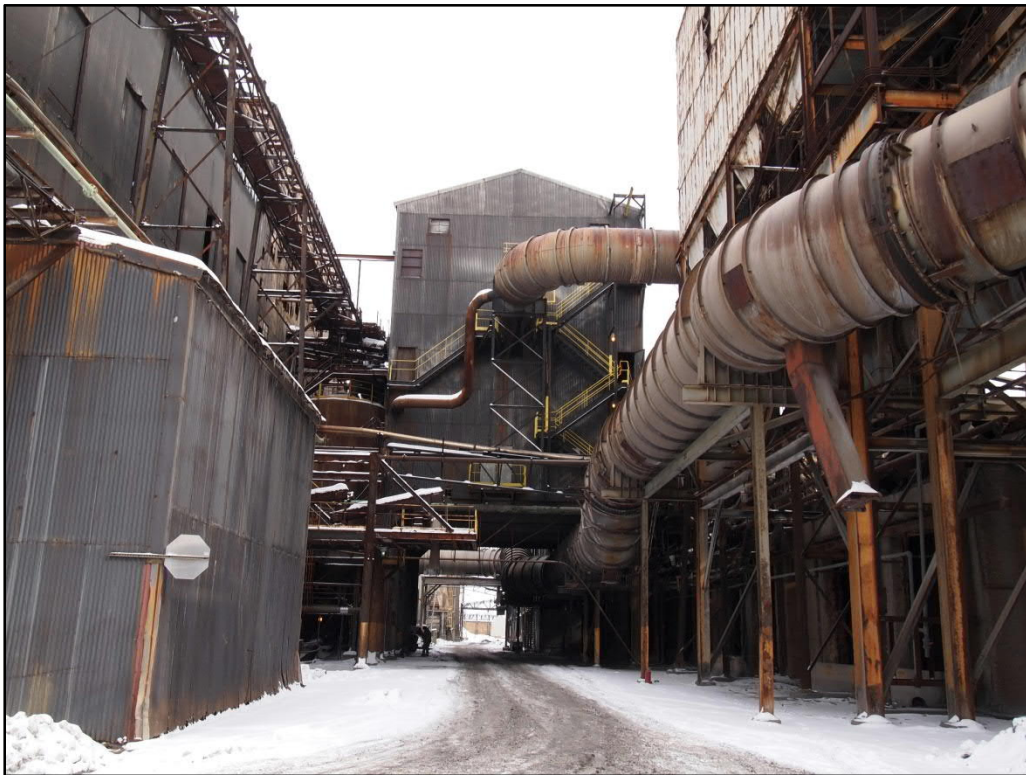
Photo 4. Bag House No. 1 (SC-3), southwest elevation, view northeast
