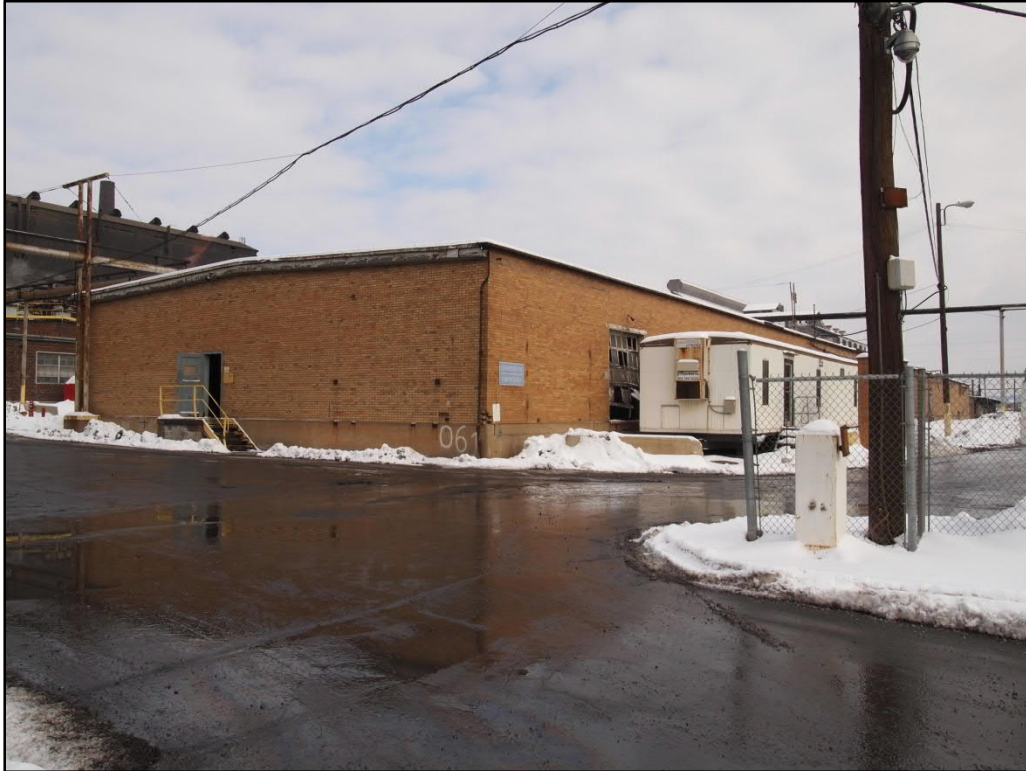
Photo 46. Zinc Oxide Storage Building (SC-33), southwest and southeast elevations, view north
