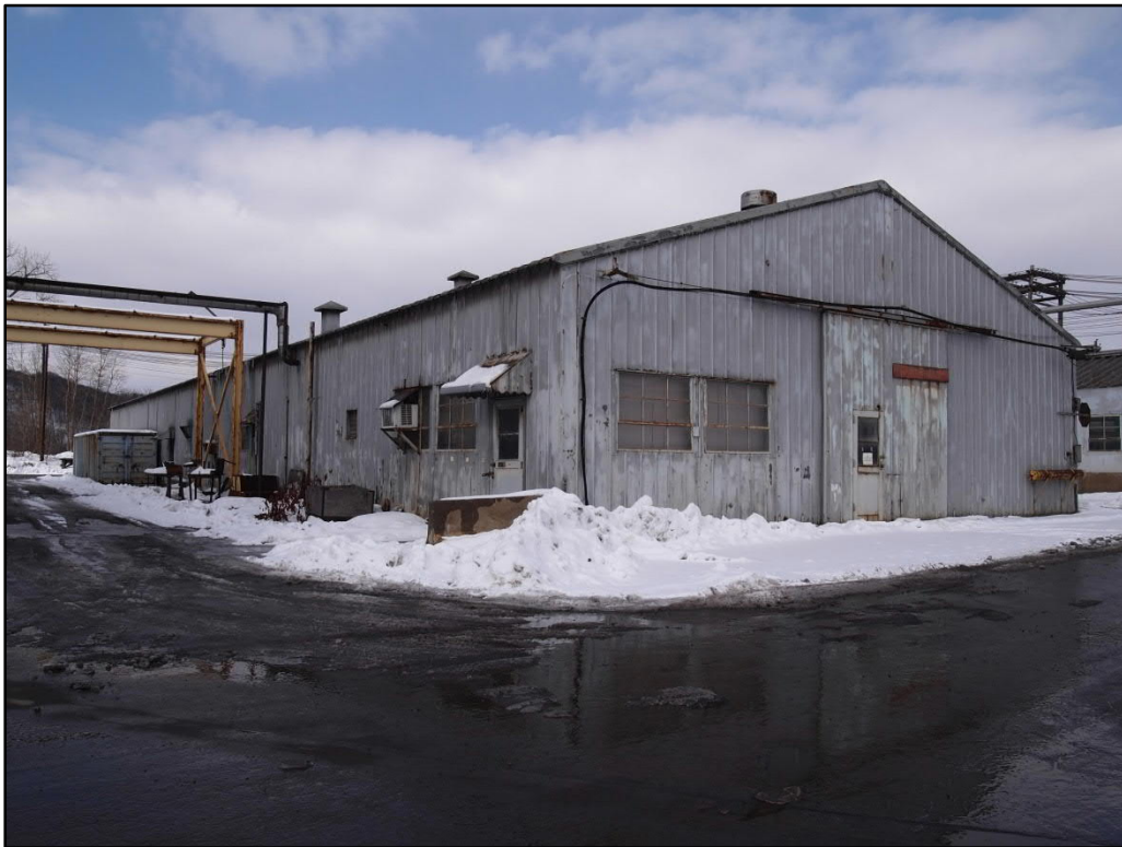
Photo 19. Heavy Maintenance Building (SC-15), front (southeast) façade and southwest elevation, view north
