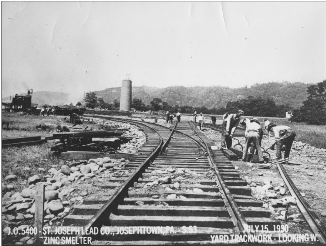
Figure 6. Yard track work and 300-foot stack under construction, July 15, 1930. 17
