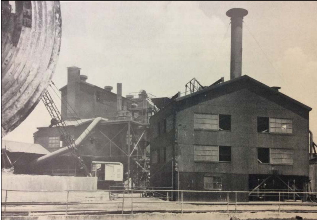
Figure 35. Secondary materials plant, 1955. 92
