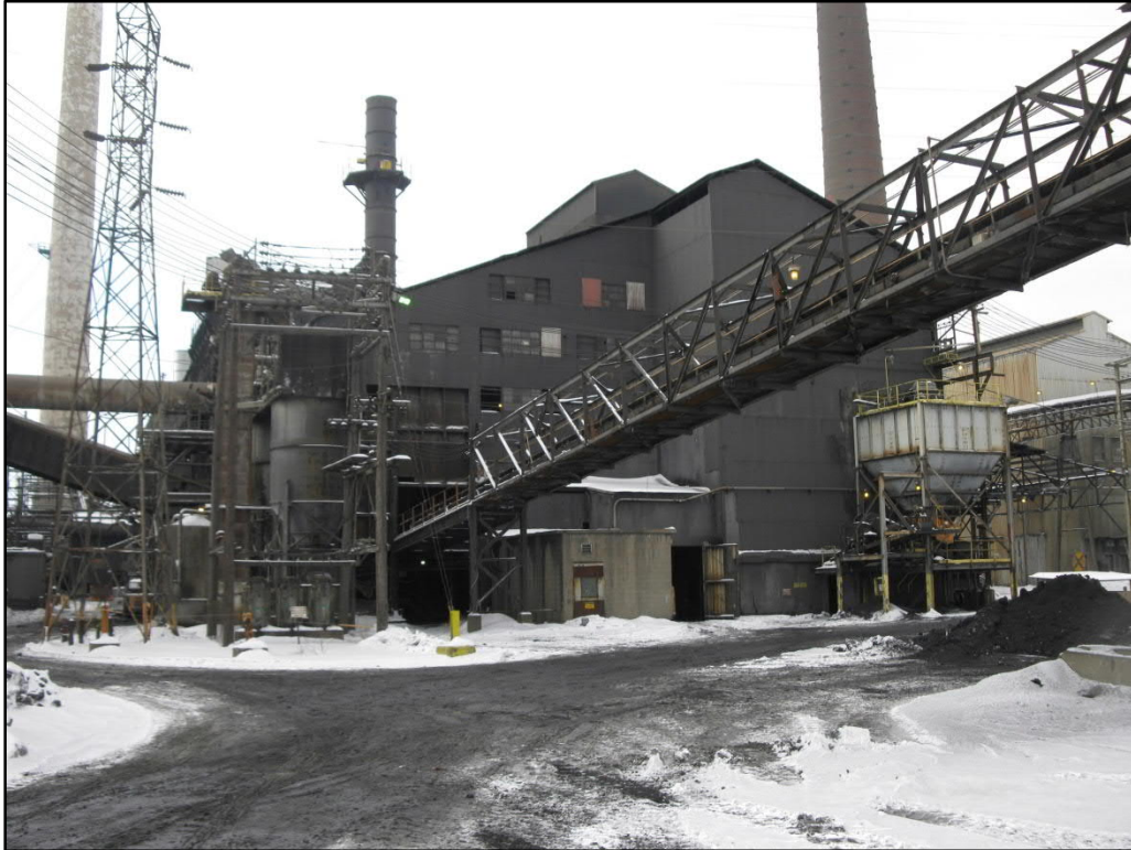
Photo 6. Coke Residue Building (SC-5), northeast elevation, view west
