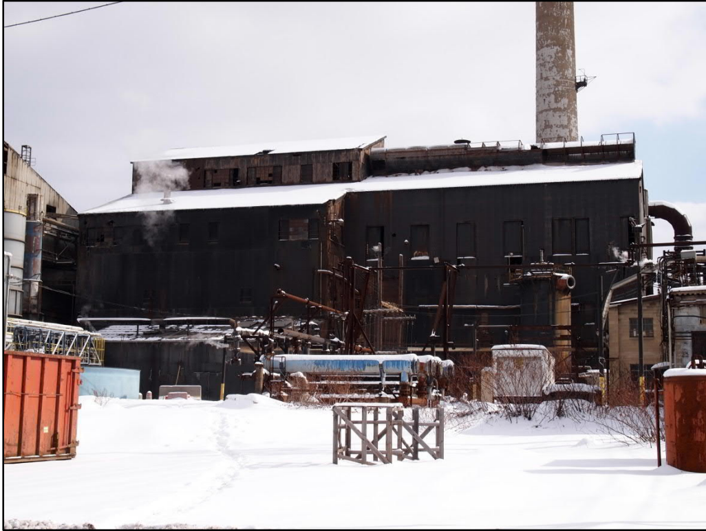
Photo 38. Roaster Plant (SC-27), northeast elevation, view southwest
