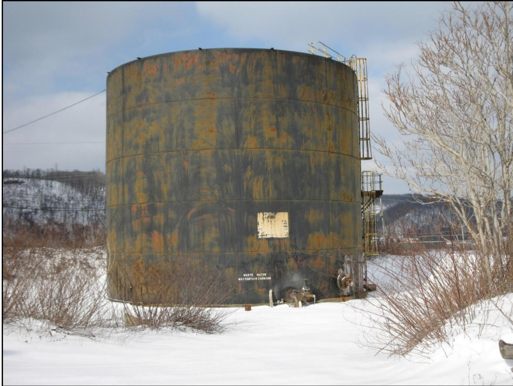
Photo 22. New Wastewater Treatment Plant (SC-18) tank, view north
