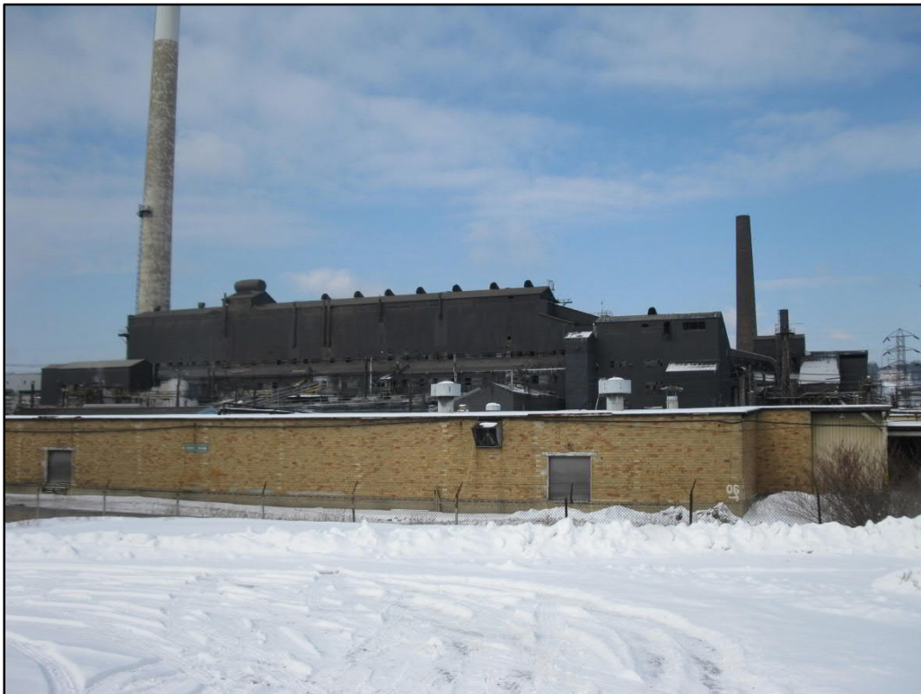
Photo 13. Furnace Plant (SC-11), southeast elevation, view northwest
