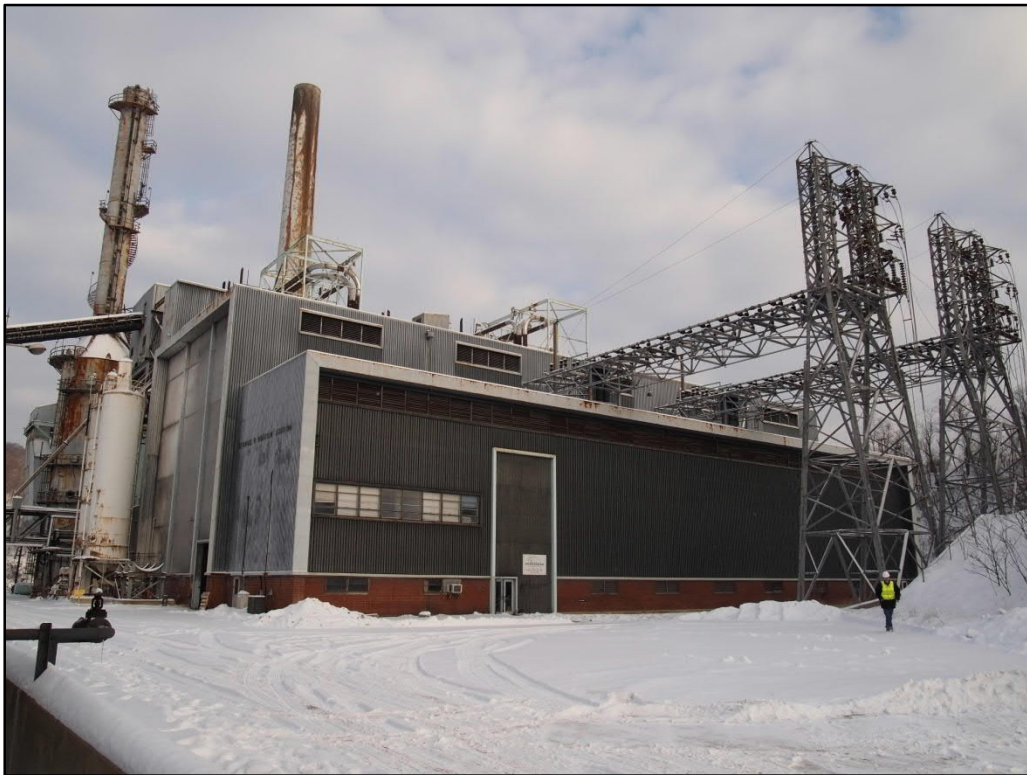
Photo 17. George F. Wheaton Power Plant (SC-13), front (southwest) facade and southeast elevation, view north
