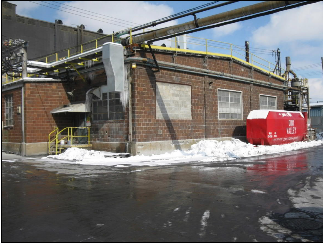
Photo 8. Compressor Building (SC-6), southeast gable end, view north
