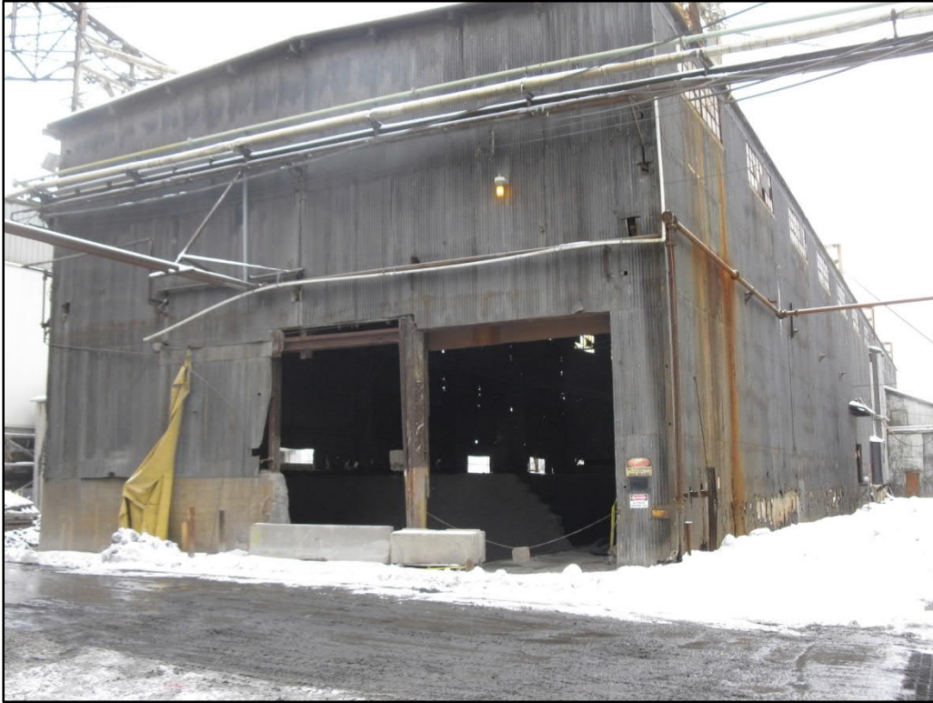
Photo 28. Ore Shed (SC-22), northeast elevation, view southwest
