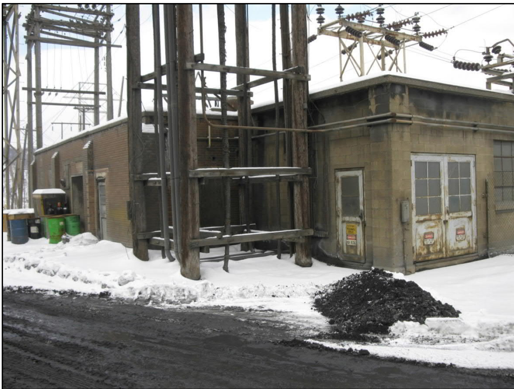
Photo 49. Old Leach Plant (SC-35), front (southwest) façade, view north
