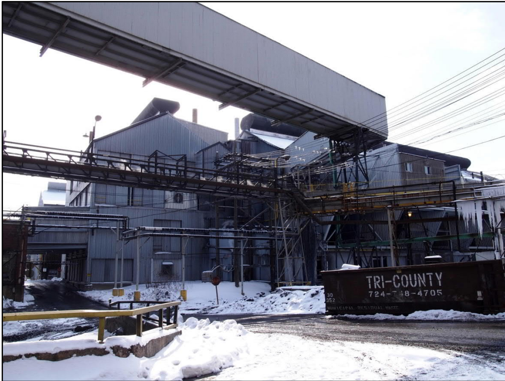
Photo 47. Zinc Refinery (SC-34), northwest elevation, view south
