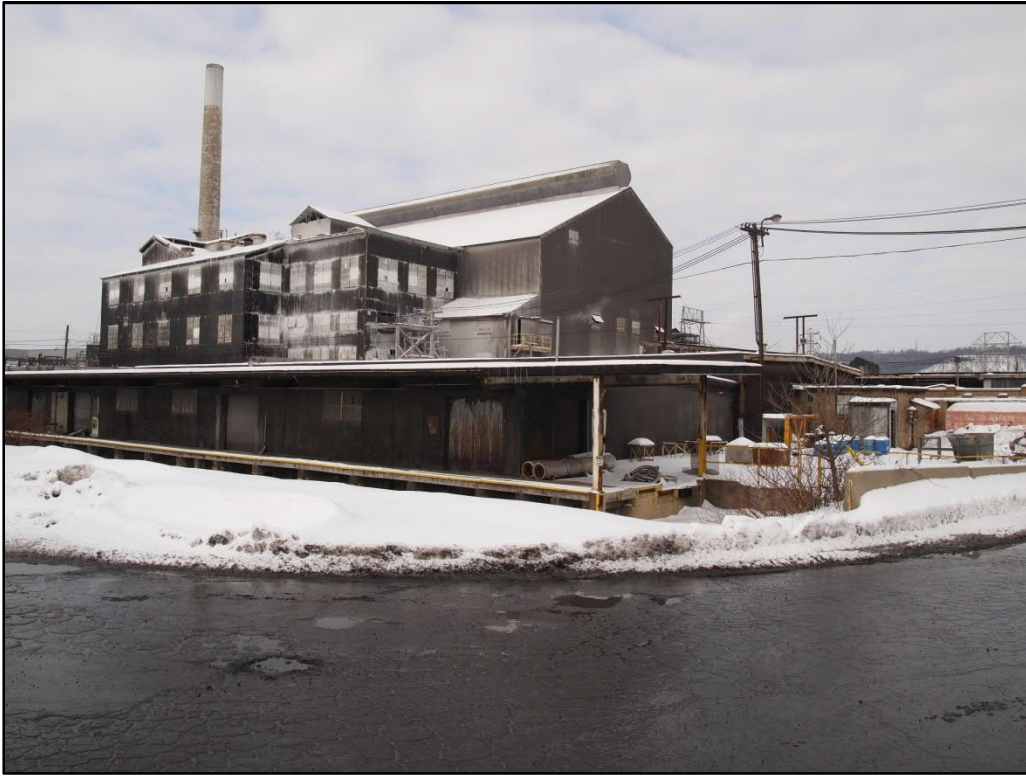
Photo 30. Oxide Department 6 (SC-23), southeast elevation, view north
