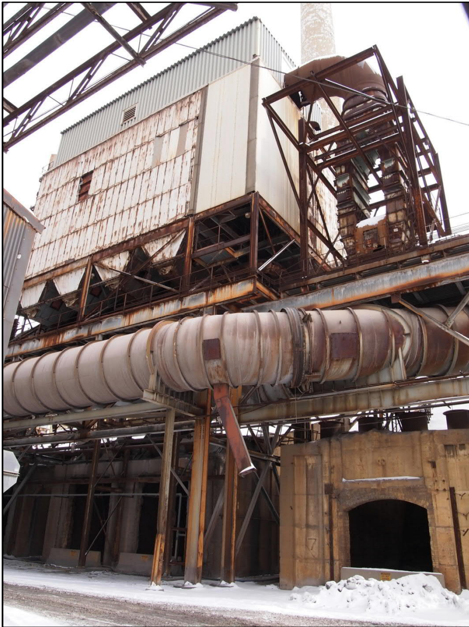
Photo 5. Bag House No. 2 (SC-4), northwest elevation, view east
