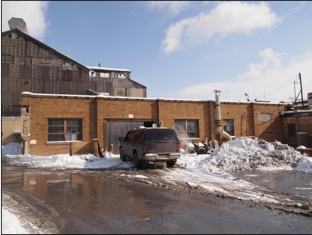
Photo 50. Cafeteria (SC-36), southwest elevation, view northeast
