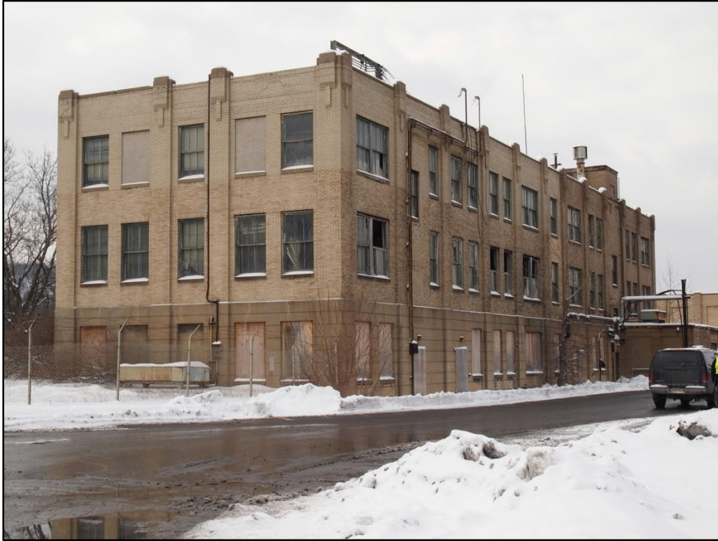
Photo 24. Old Main Office (SC-19), rear (northwest) and southeast elevations, view south
