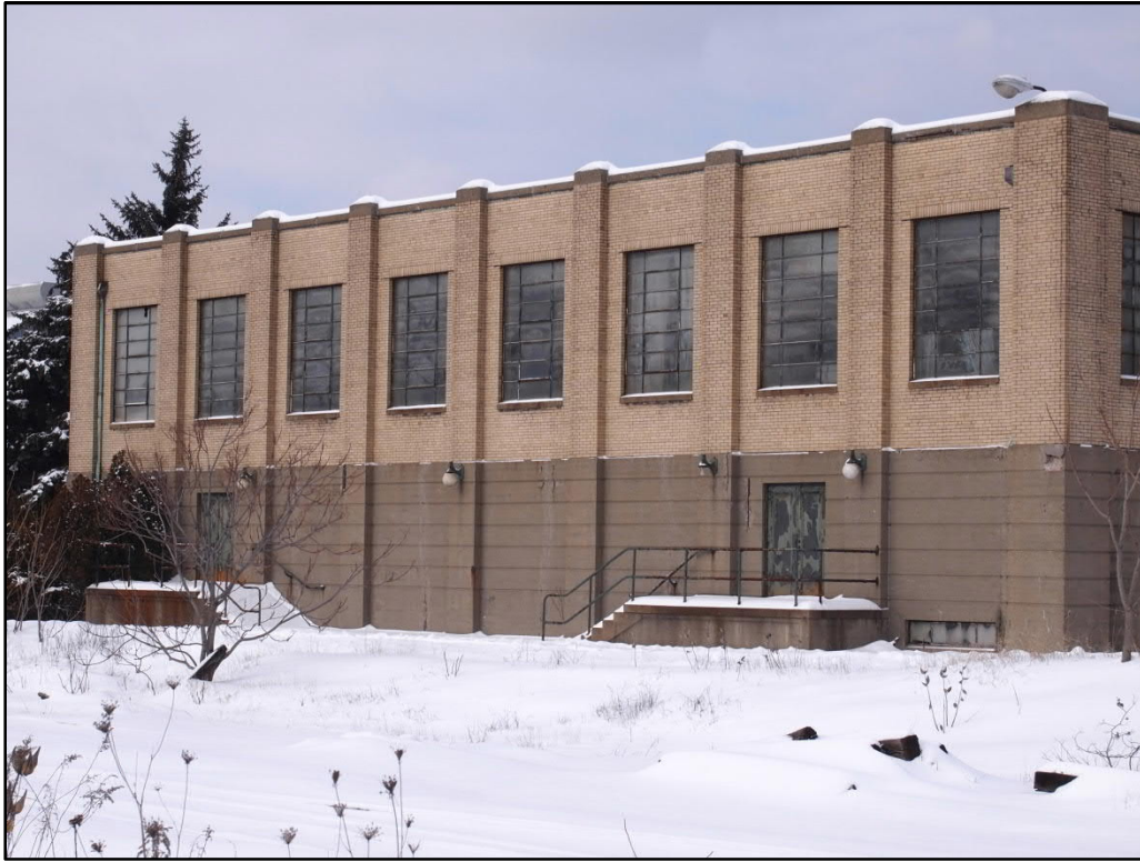
Photo 18. Auditorium (SC-14), front (southeast) façade, view west
