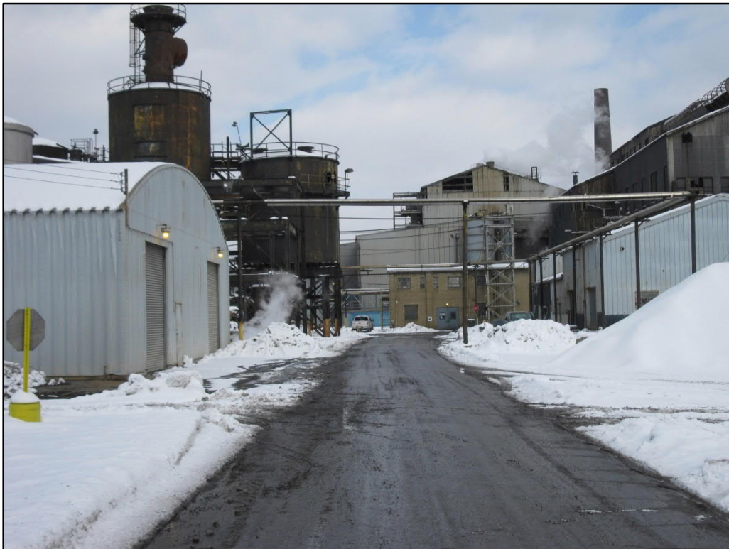
Photo 21. Motor (West) Storage Building (SC-17) [right side of image], view northeast
