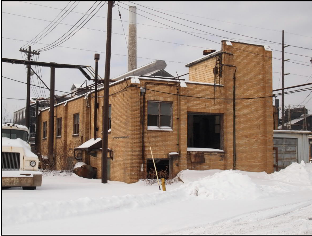
Photo 26. Wet Lab (SC-20), rear (northeast) elevation, view west
