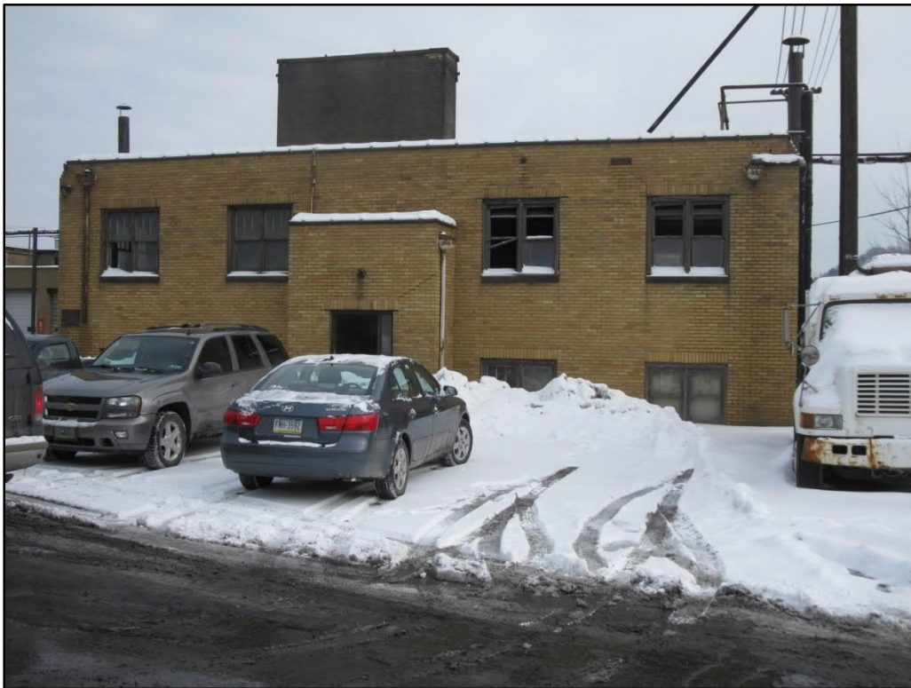
Photo 25. Wet Lab (SC-20), front (southwest) elevation, view northeast
