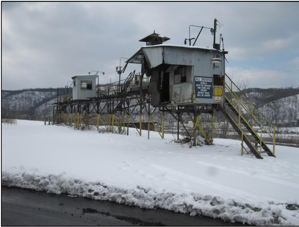
Photo 1. Acid Loading Rack (SC-1), view west
