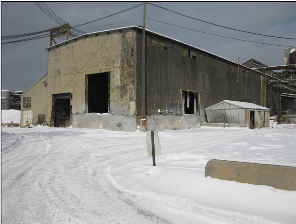
Photo 29. Ore Shed (SC-22), southwest and southeast elevations, view north
