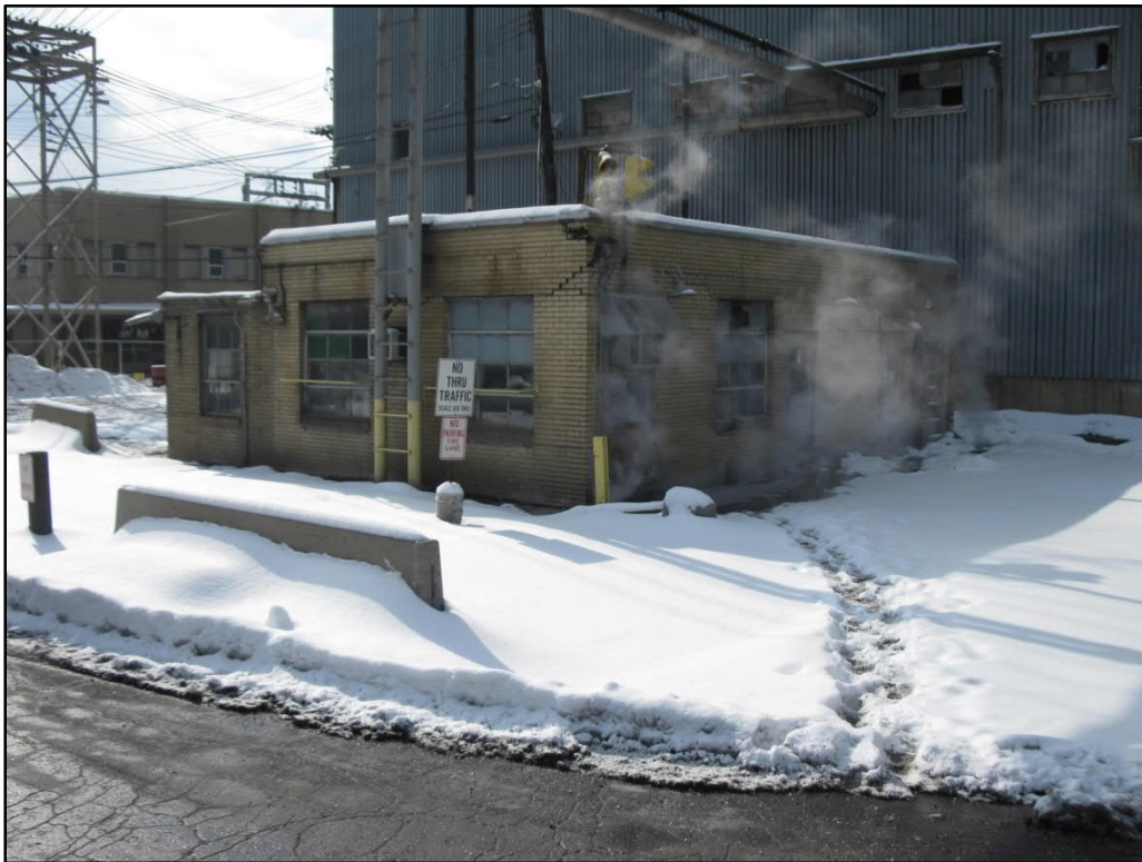
Photo 51. Scale House (SC-37), northwest and northeast elevations, view south
