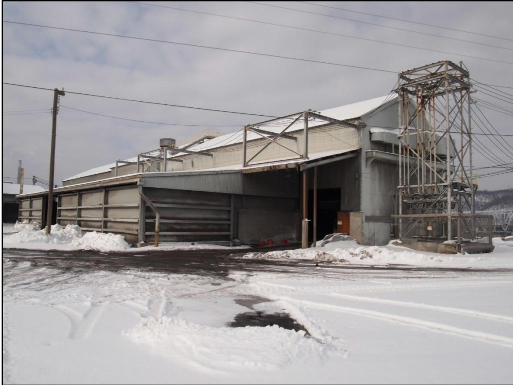
Photo 40. Secondary Materials Storage (SC-29), northeast and southeast elevations, view west
