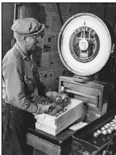
Figure 27. Weighing cadmium balls in the leach plant. 77
