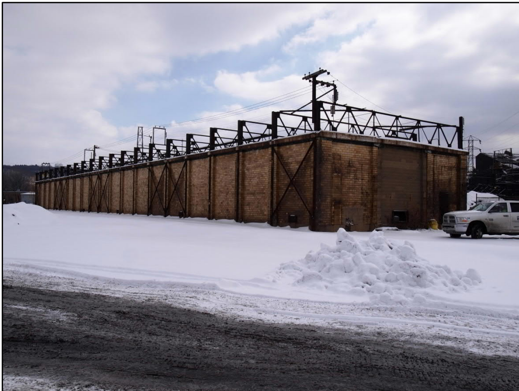
Photo 27. Old Thaw House (SC-21), northwest and northeast elevations, view south
