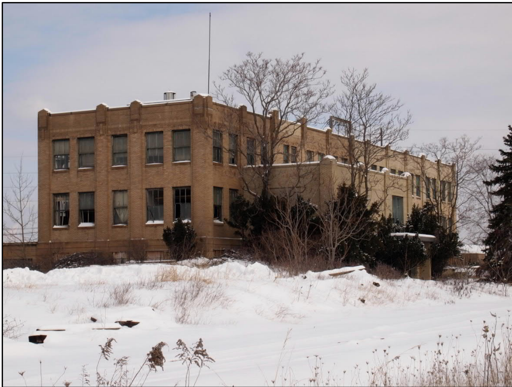
Photo 23. Old Main Office (SC-19), front (southeast) façade and southwest elevation, view north
