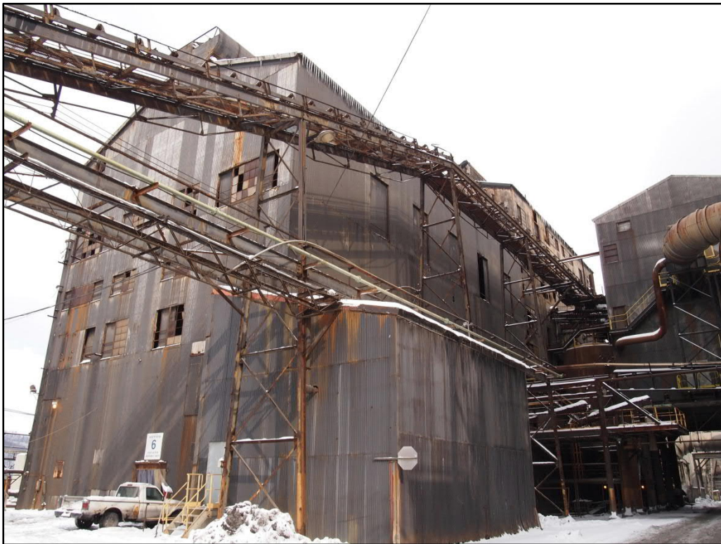
Photo 37. Roaster Plant (SC-27), southwest and southeast elevations, view north
