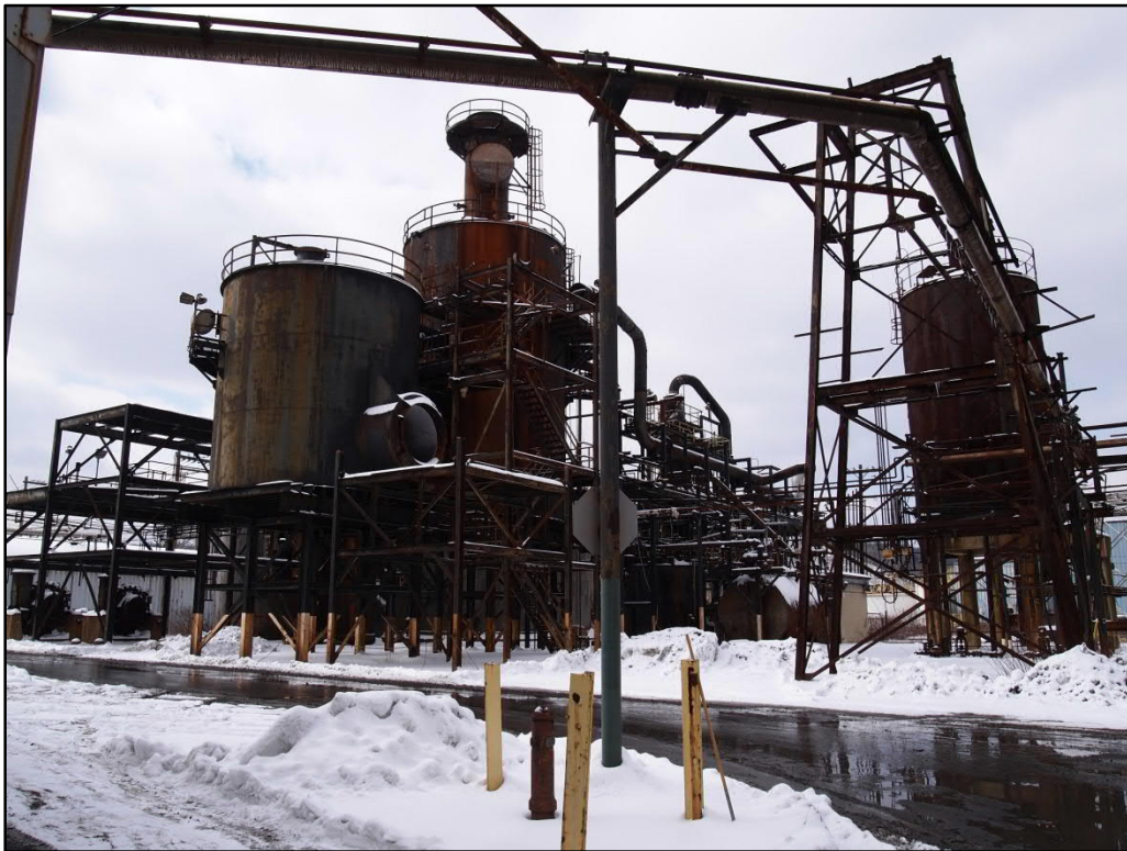
Photo 2. Old Acid Plant (SC-2), view south
