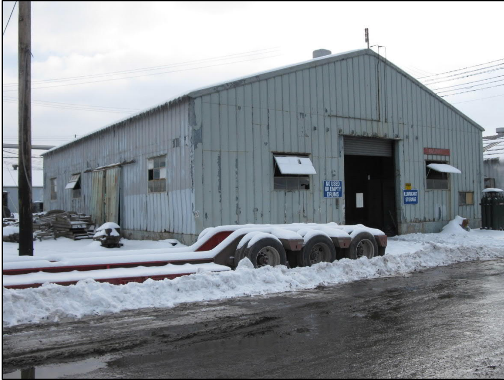
Photo 20. Lubricant Storage Building (SC-16), front (northwest) façade and northeast elevation, view south
