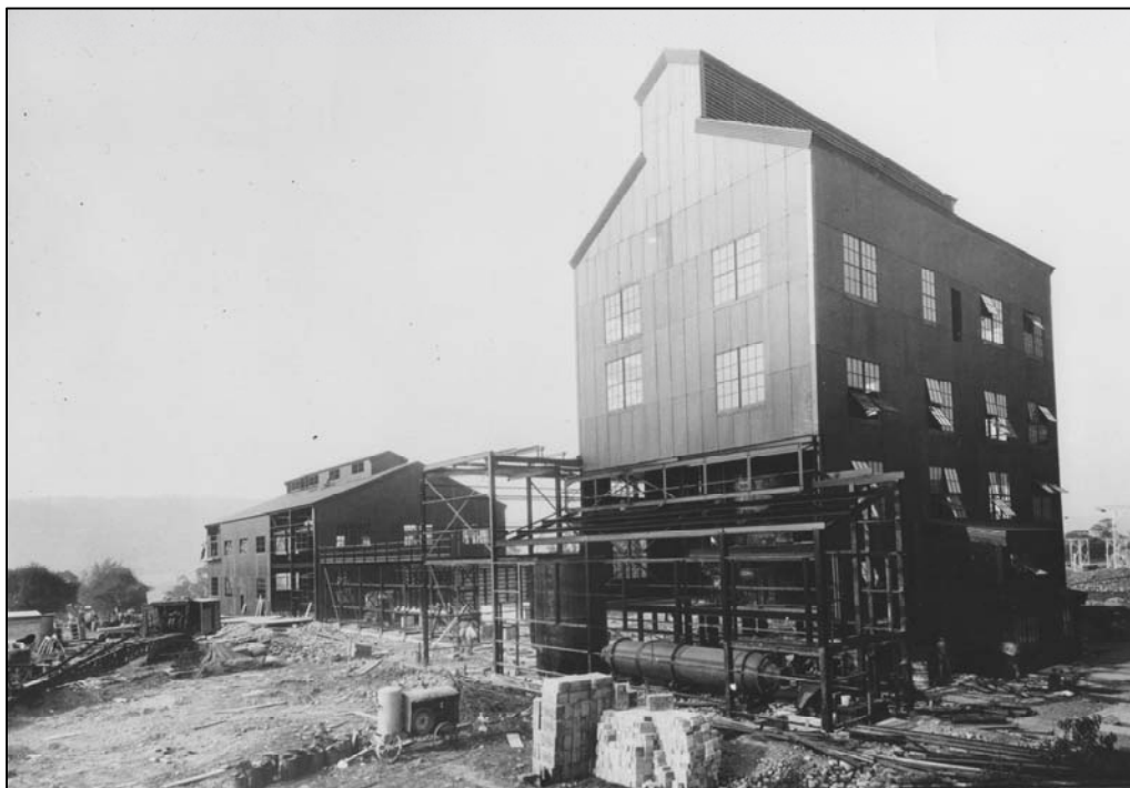
Figure 8. Acid plant (left) and roaster plant (right) under construction, September 18, 1930. 18
