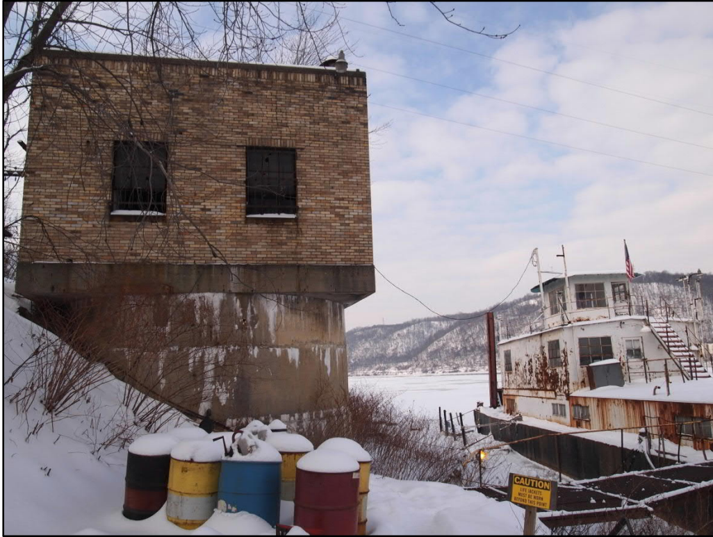
Photo 36. Pump House No. 1 (SC-26), side (northeast) elevation and Ohio River, view west
