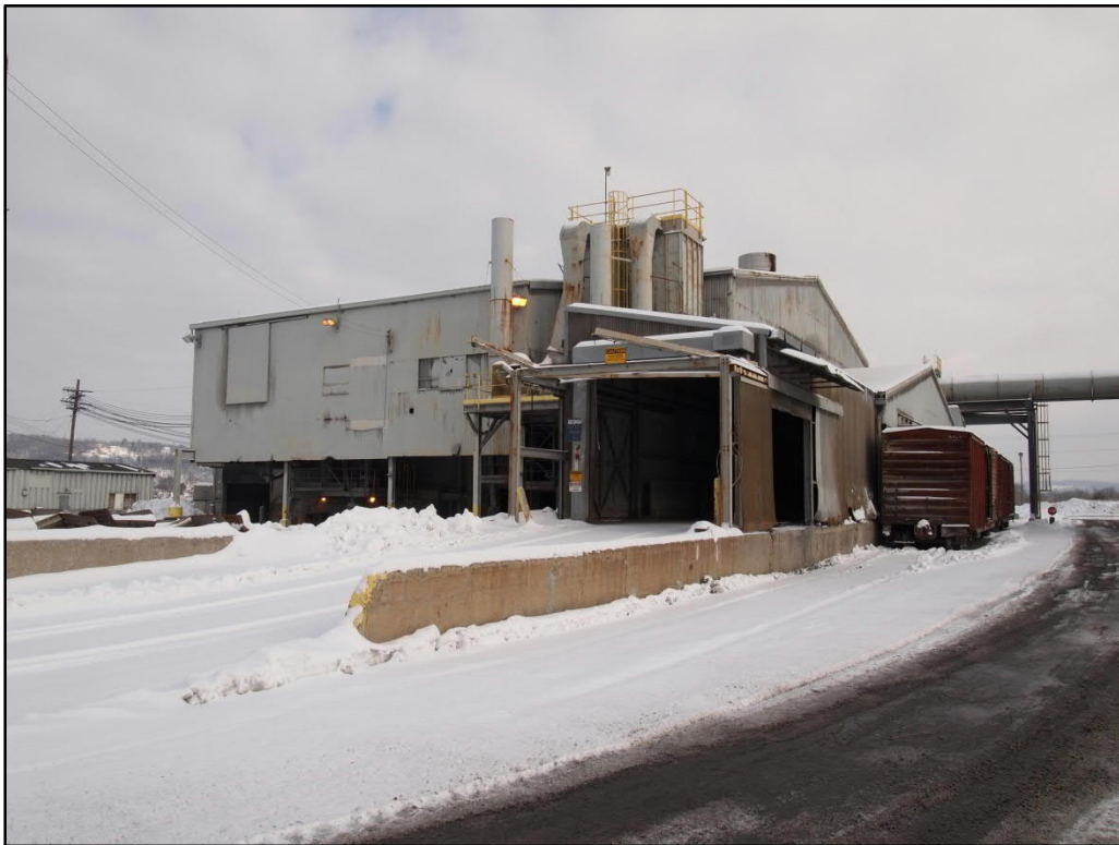
Photo 39. Secondary Materials Plant (SC-28), southeast and southwest elevations, view north
