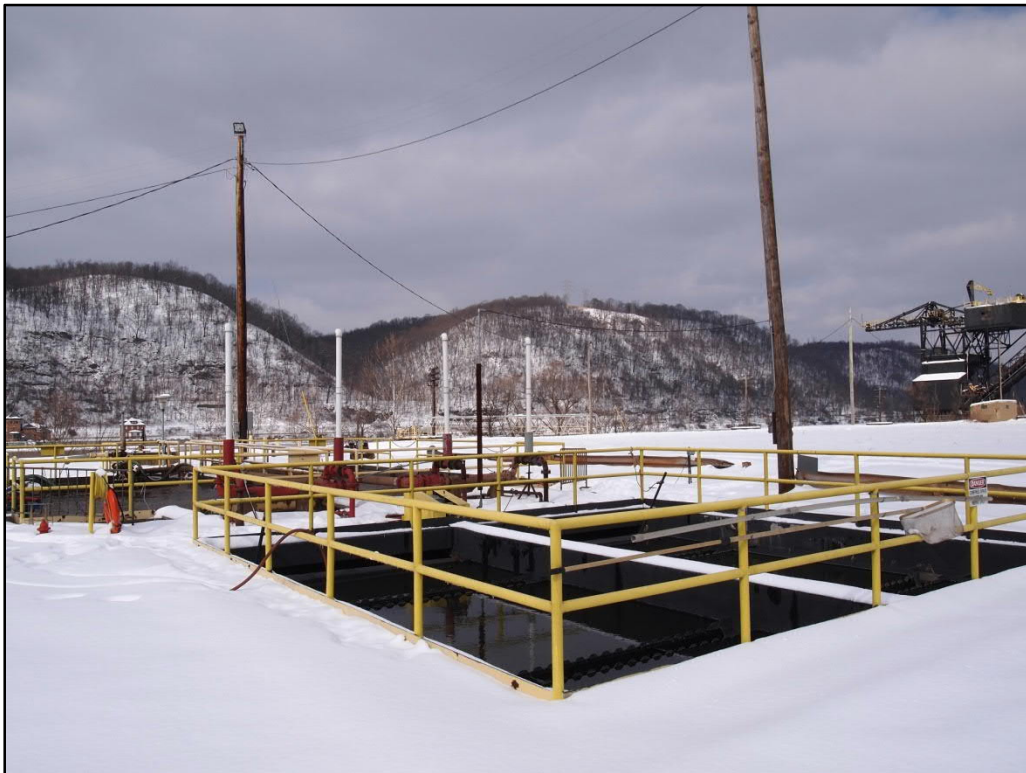
Photo 43. Power Plant Treatment/Sewage Plant (SC-31), Wastewater pool, view northeast
