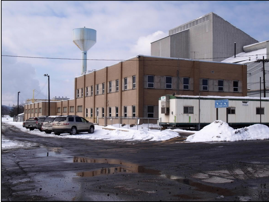
Photo 32. Personnel Building (SC-24), front (northeast) façade and southeast elevation, view west
