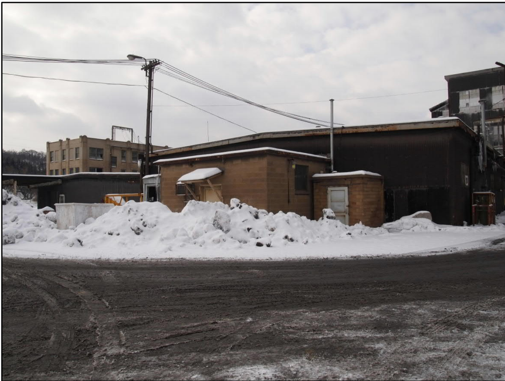
Photo 31. Oxide Department 6 (SC-23), northeast elevation, view southwest
