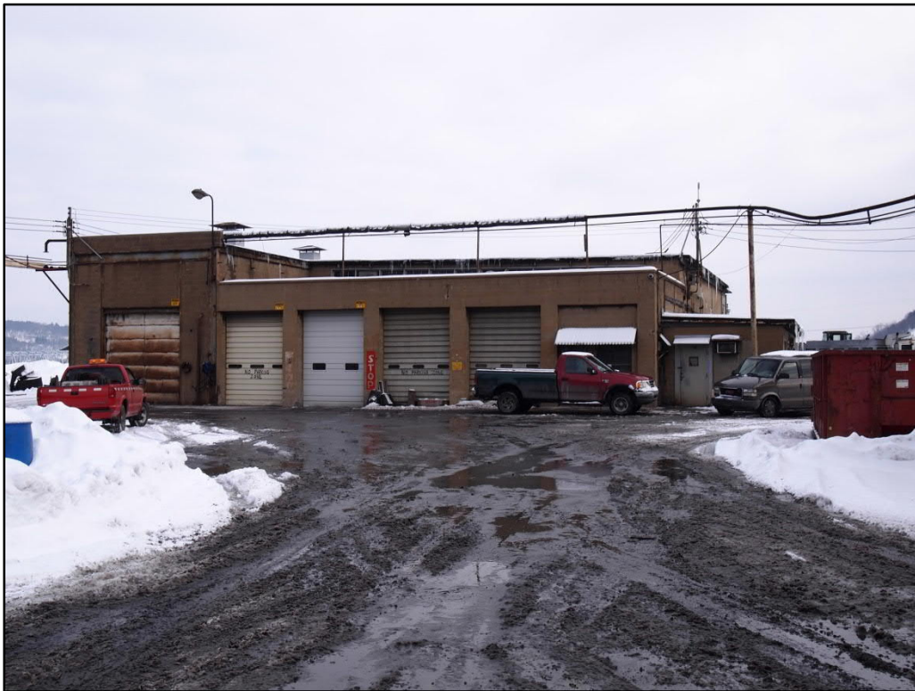
Photo 15. Garage (SC-12), front (southwest) façade, view northeast
