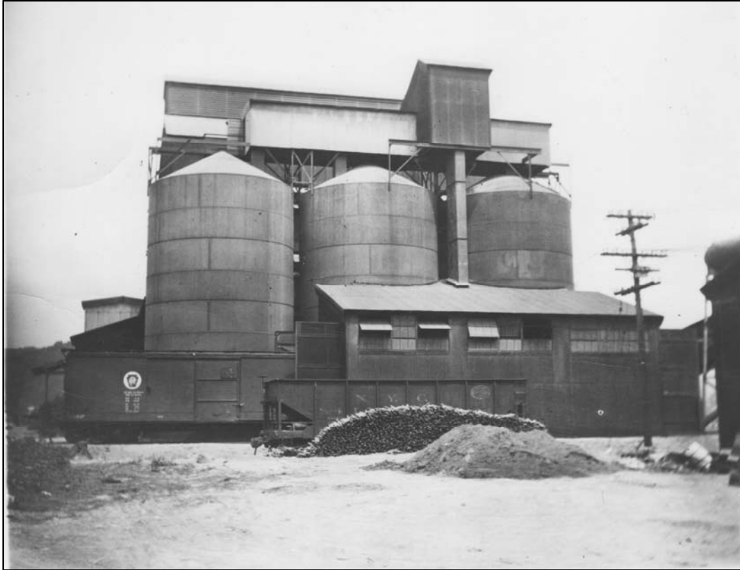
Figure 21. Ore storage bins at the roaster plant. 59
