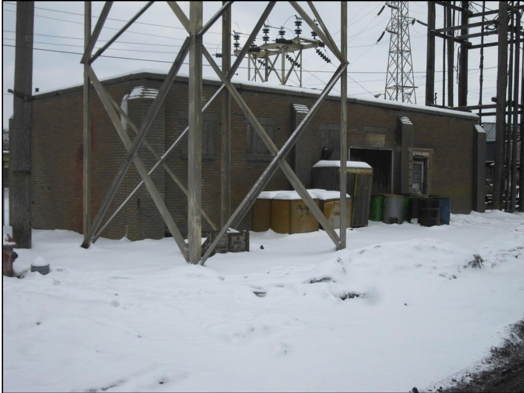
Photo 48. Old Leach Plant (SC-35), front (southwest) façade, view northeast
