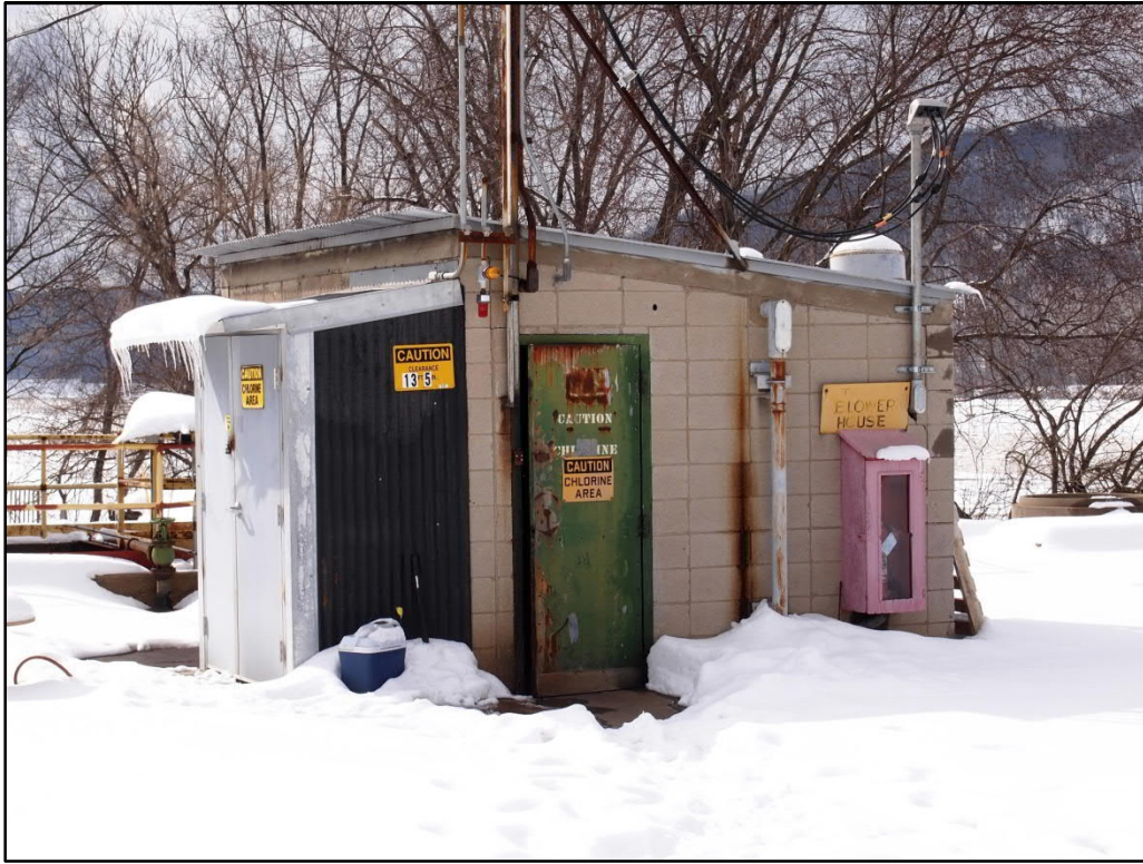
Photo 42. Power Plant Treatment/Sewage Plant (SC-31), Blower House, view west
