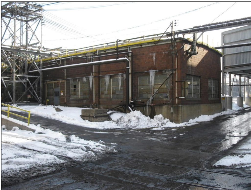
Photo 7. Compressor Building (SC-6), northwest elevation, view east
