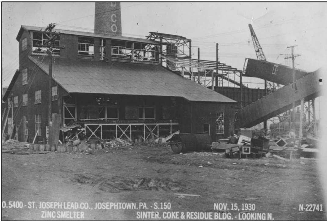
Figure 12. Construction of the sinter, coke and residue building, November 15, 1930. 21
