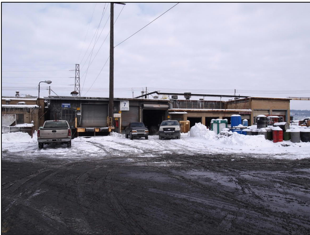
Photo 41. Store Room No. 1 (SC-30), southeast elevation, view northwest
