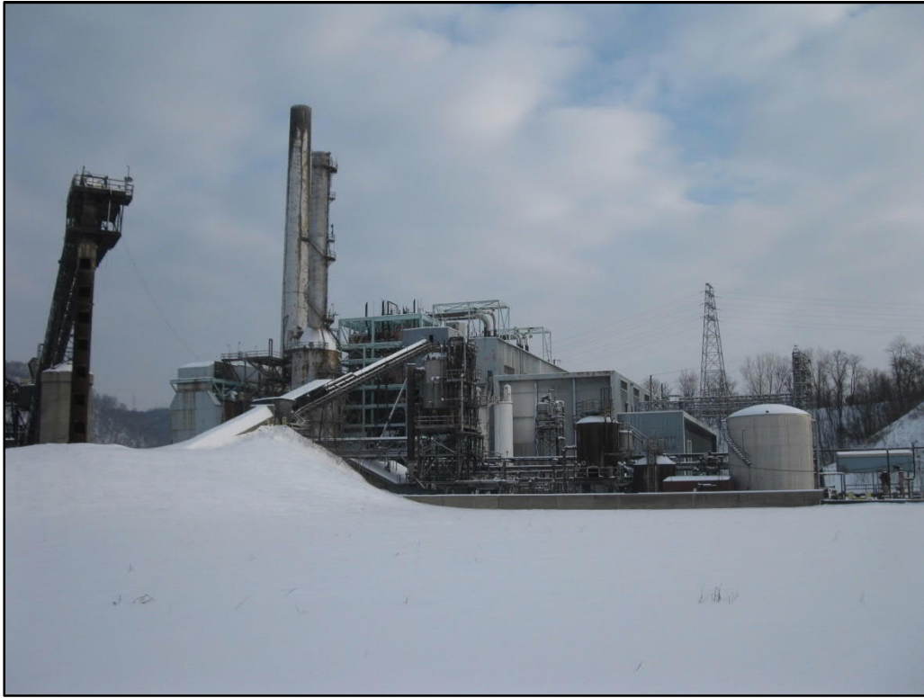
Photo 16. George F. Wheaton Power Plant (SC-13), view north
