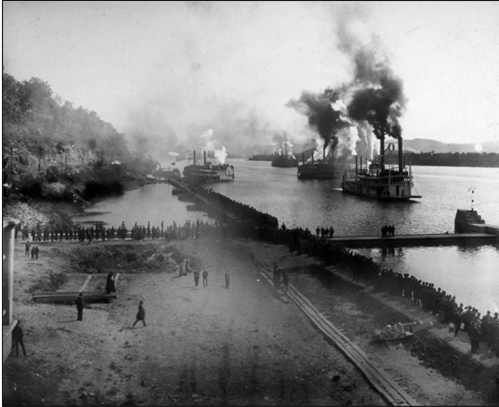
Figure 6. Davis Island Lock and Dam opening celebrations, October 7, 1885. 63
