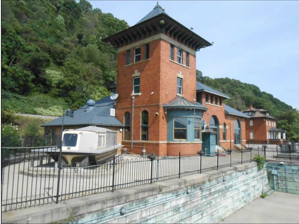
Photo 1. Merrill Lock No. 6. View north of former powerhouse.
