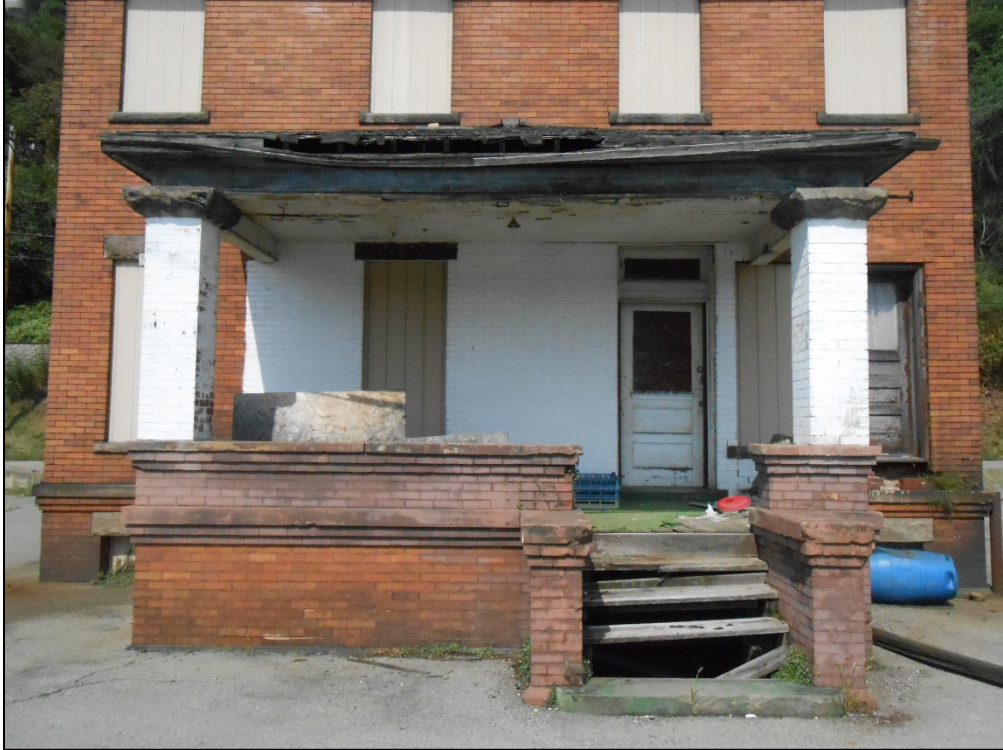
Photo 9. Merrill Lock No. 6. Detail view of front façade of former lockkeeper's house.
