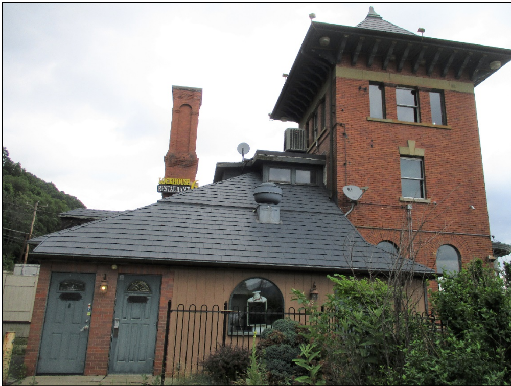
Photo 4. Merrill Lock No. 6. Detail view of southwest façade.
