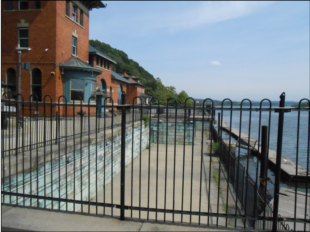
Photo 5. Merrill Lock No. 6. View northeast of esplanade.
