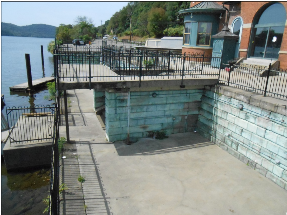
Photo 6. Merrill Lock No. 6. View southwest of esplanade.
