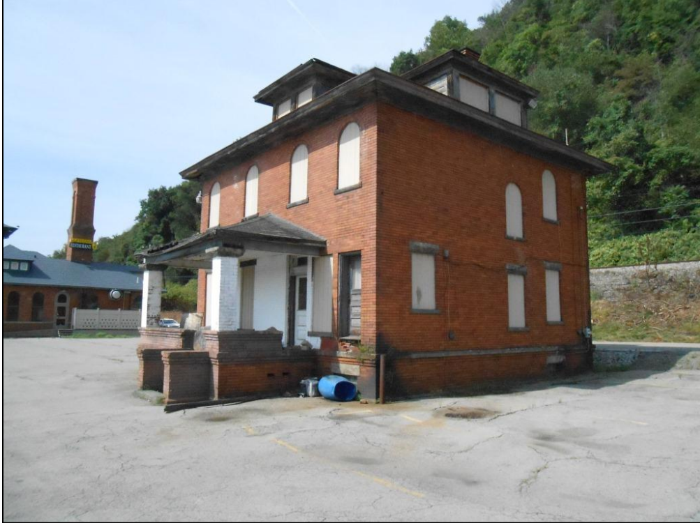
Photo 7. Merrill Lock No. 6. View southwest of former lockkeeper's house.
