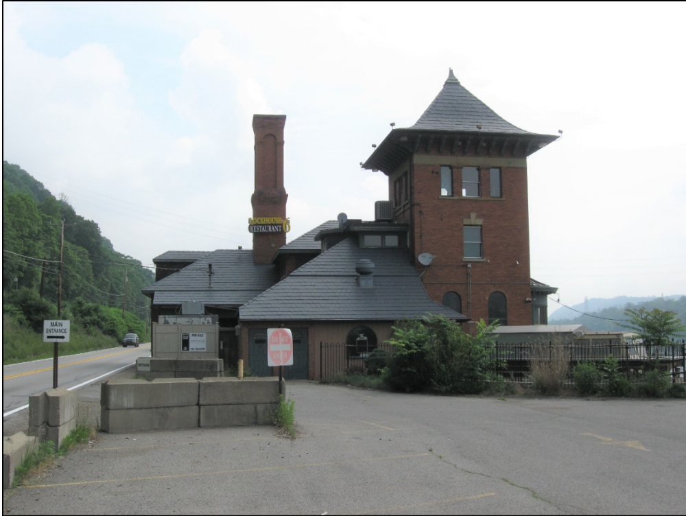
Photo 3. Merrill Lock No. 6. View northeast of former powerhouse.
