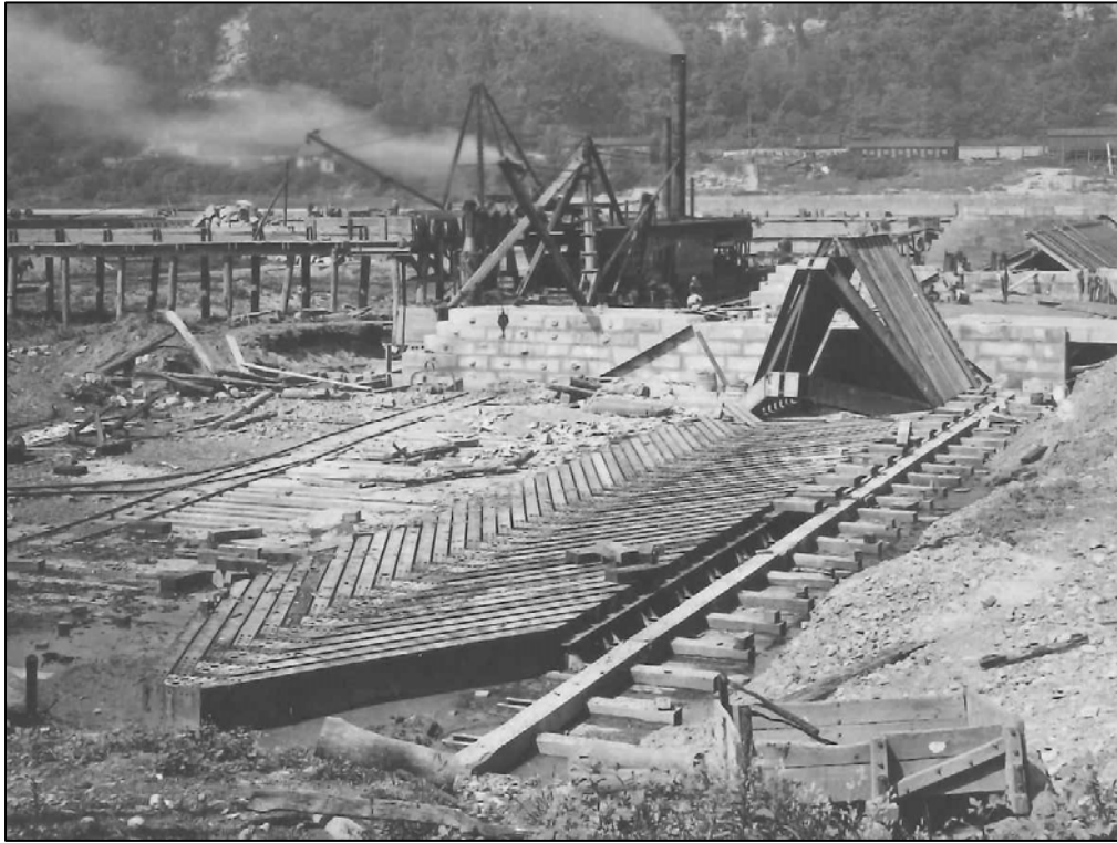
Figure 13. Thomas A-frame dam at Merrill Lock and Dam No. 6. 107
