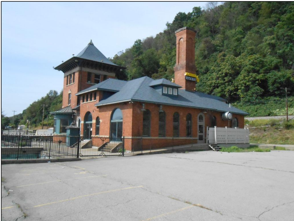
Photo 2. Merrill Lock No. 6. View southwest of former powerhouse.
