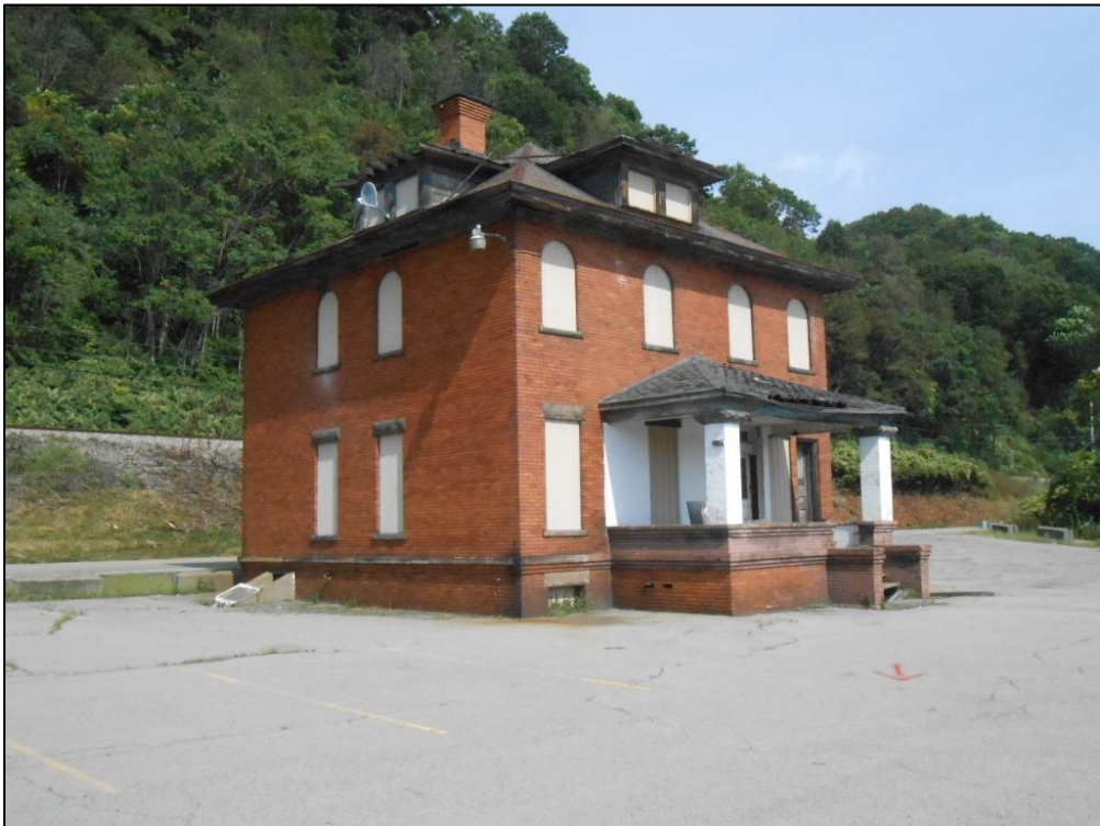
Photo 8. Merrill Lock No. 6. View north of former lockkeeper's house.
