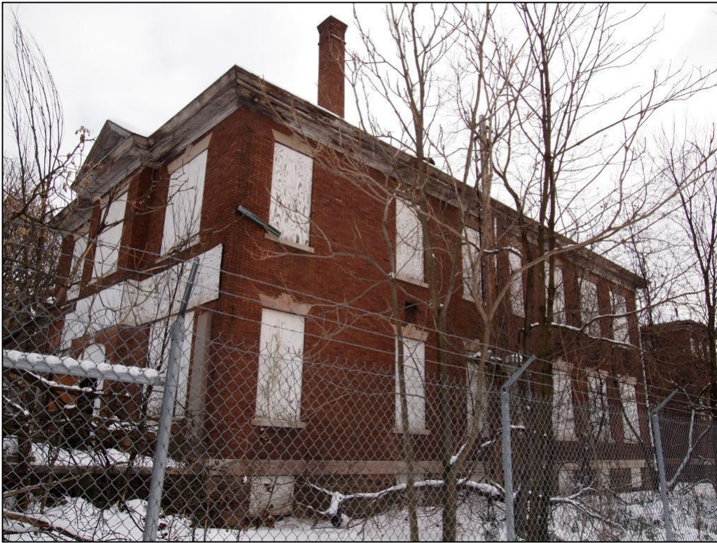
13. Beaver County Home. View east of side façade of west wing.
