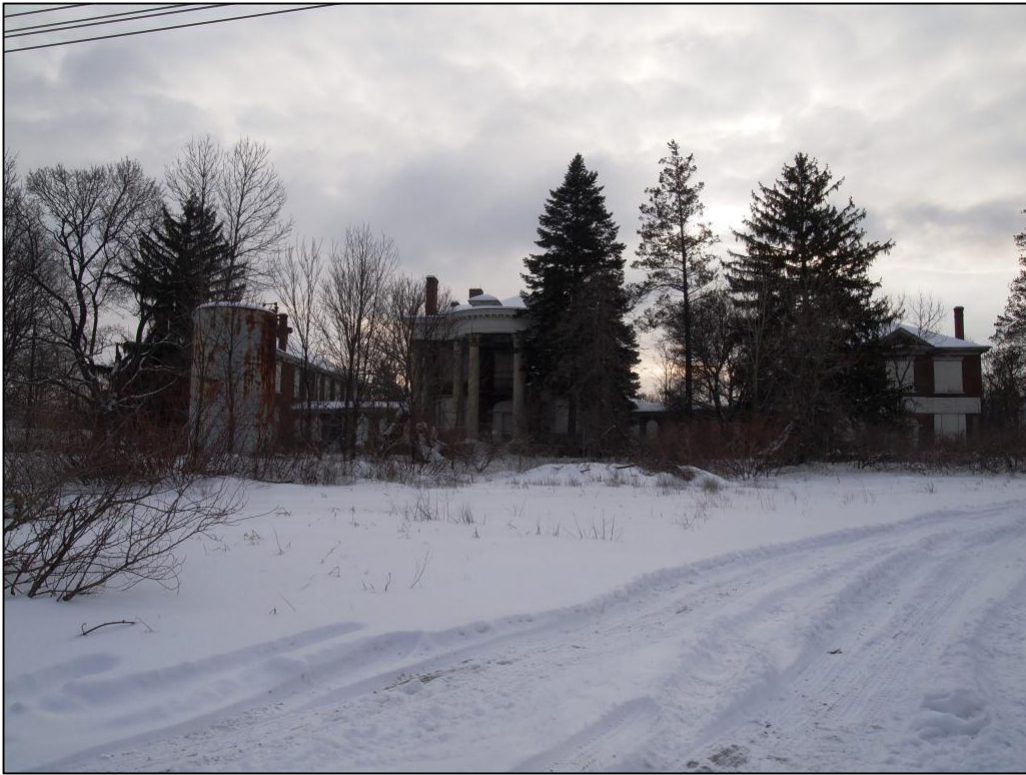
1. Beaver County Home. View southeast of front façade.
