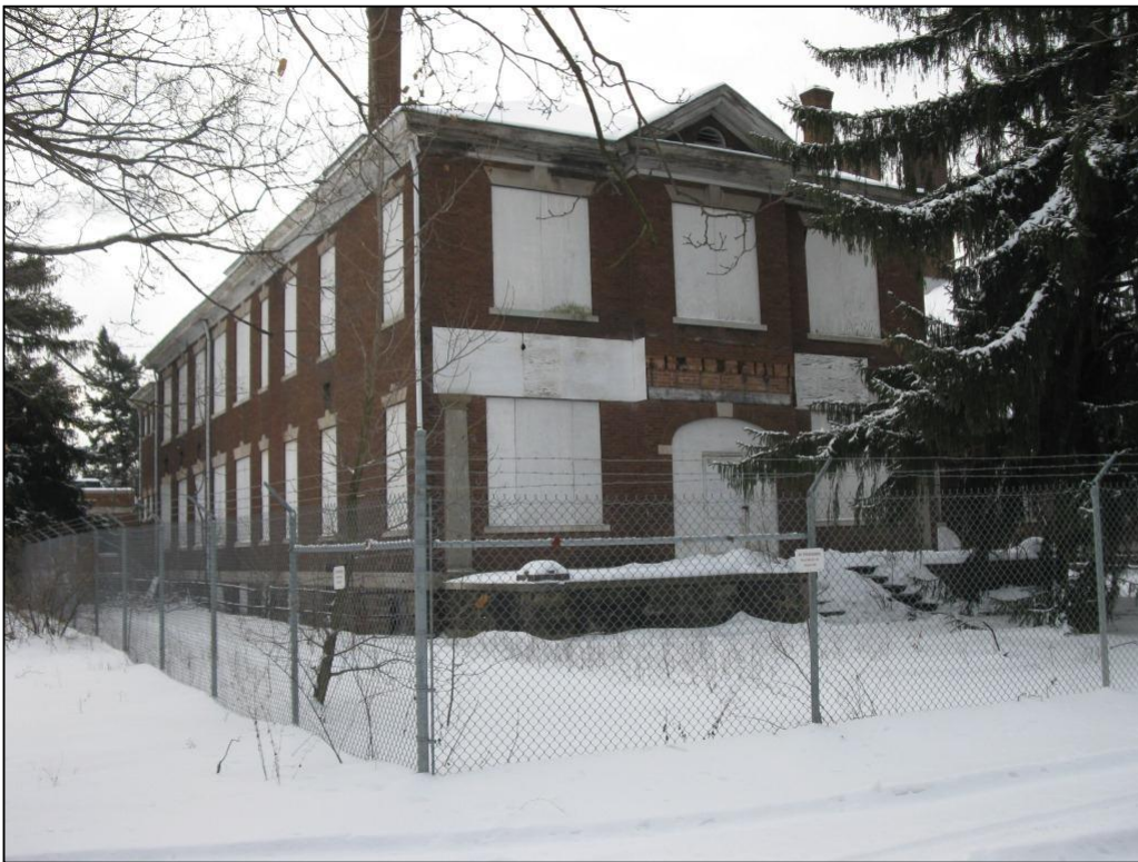
8. Beaver County Home. View south of front façade of east wing.
