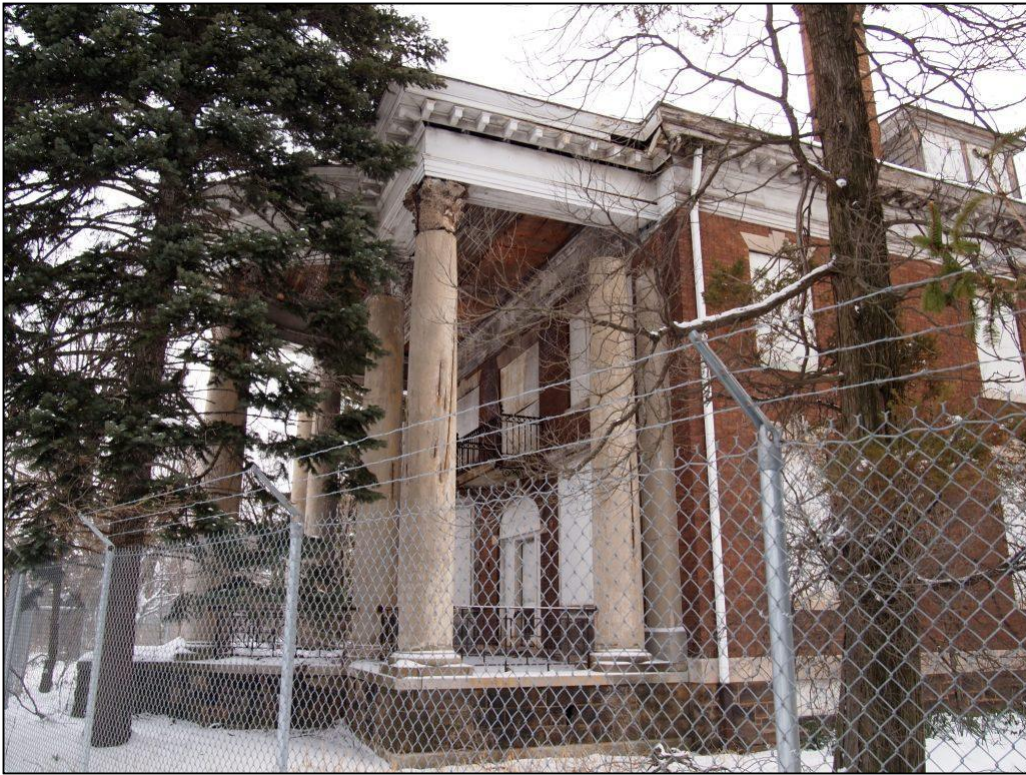
3. Beaver County Home. View northeast of front portico.
