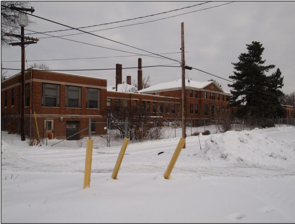
19. Beaver County Home. View north of 1940 addition.
