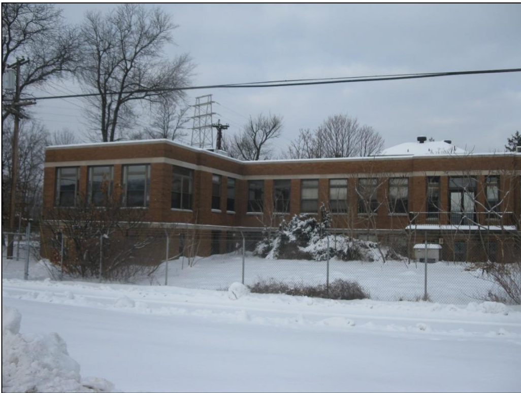
18. Beaver County Home. View northwest of western half of 1940 addition.
