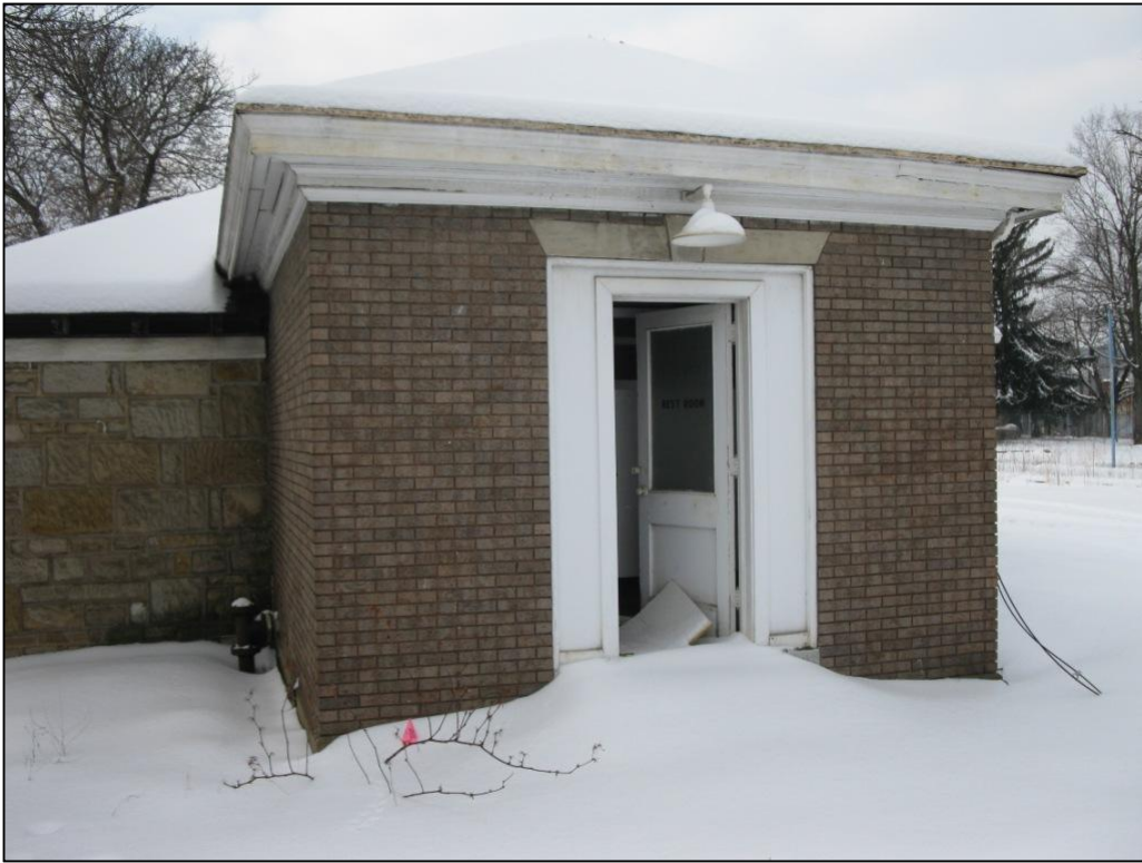
23. Beaver County Home. View west of outdoor pavilion.
