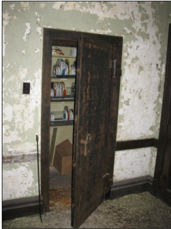
31. Beaver County Home. View of vault in former main office.
