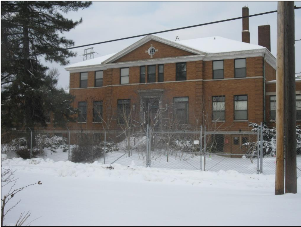
17. Beaver County Home. View northwest of entranceway of 1940 addition.
