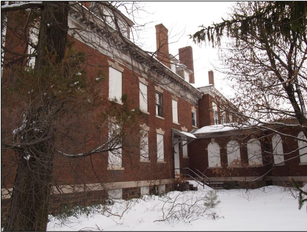
11. Beaver County Home. View east of side façade of central building.
