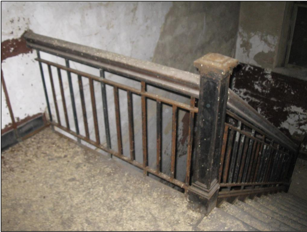
37. Beaver County Home. View of stairwell in east wing.
