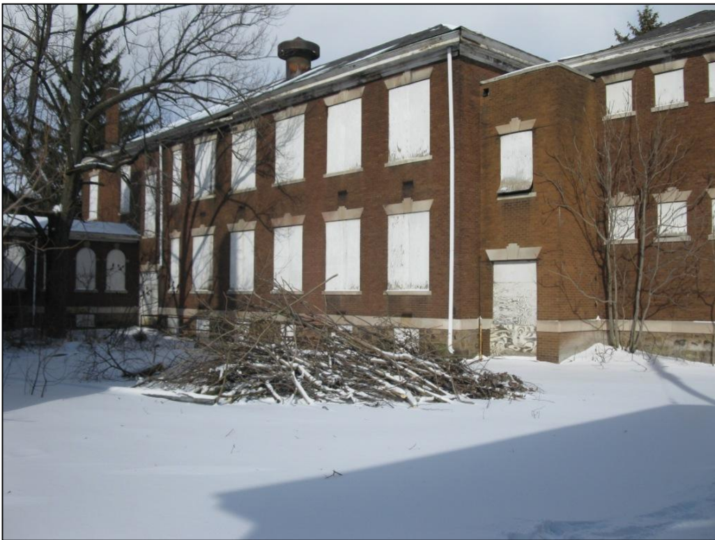
16. Beaver County Home. View north of courtyard façade of east wing.
