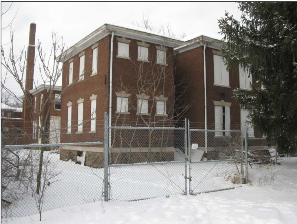
10. Beaver County Home. View west of rear façade of east wing.
