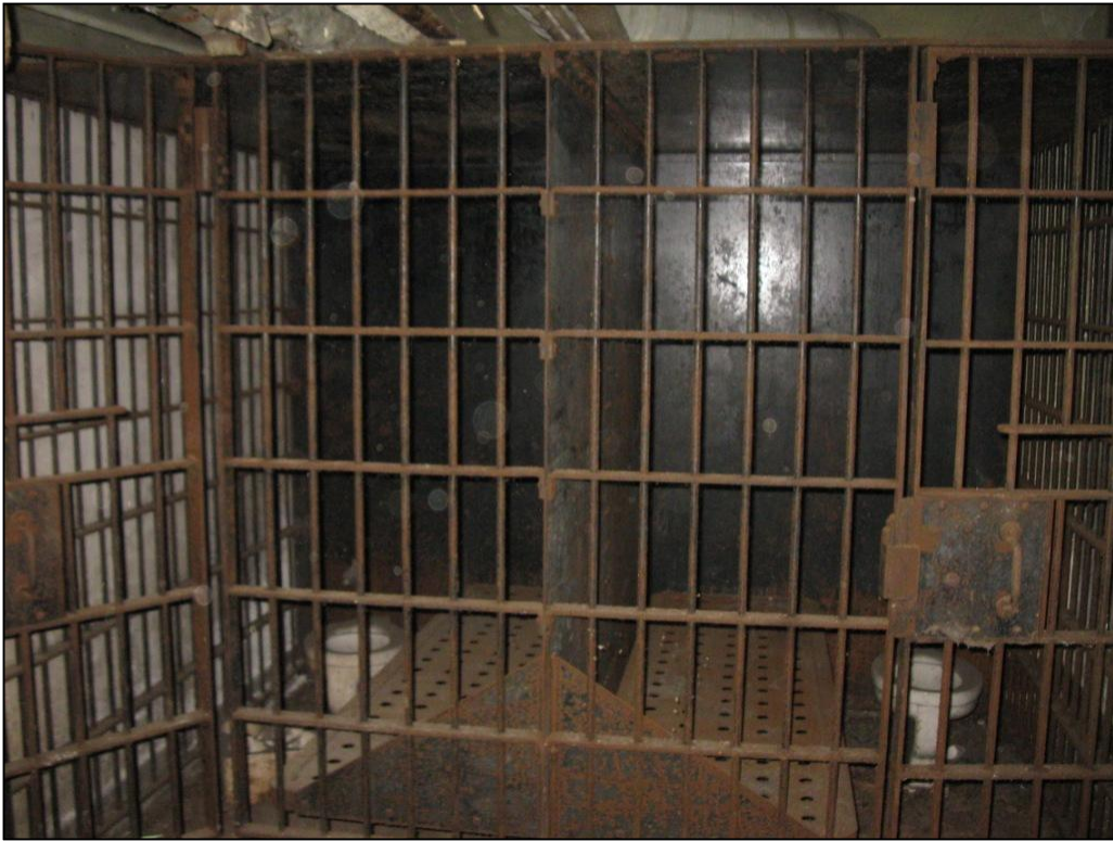
33. Beaver County Home. View of portable jail cell in basement of central building.
