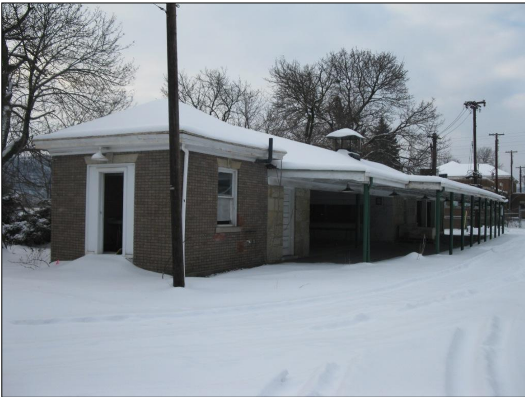
22. Beaver County Home. View southwest of outdoor pavilion.
