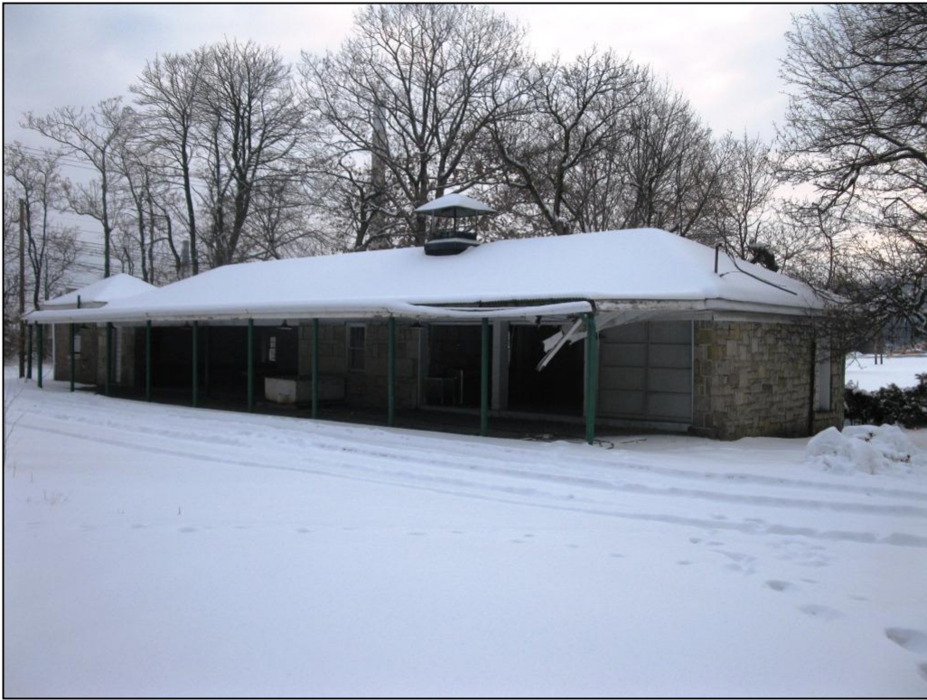
21. Beaver County Home. View east of outdoor pavilion.
