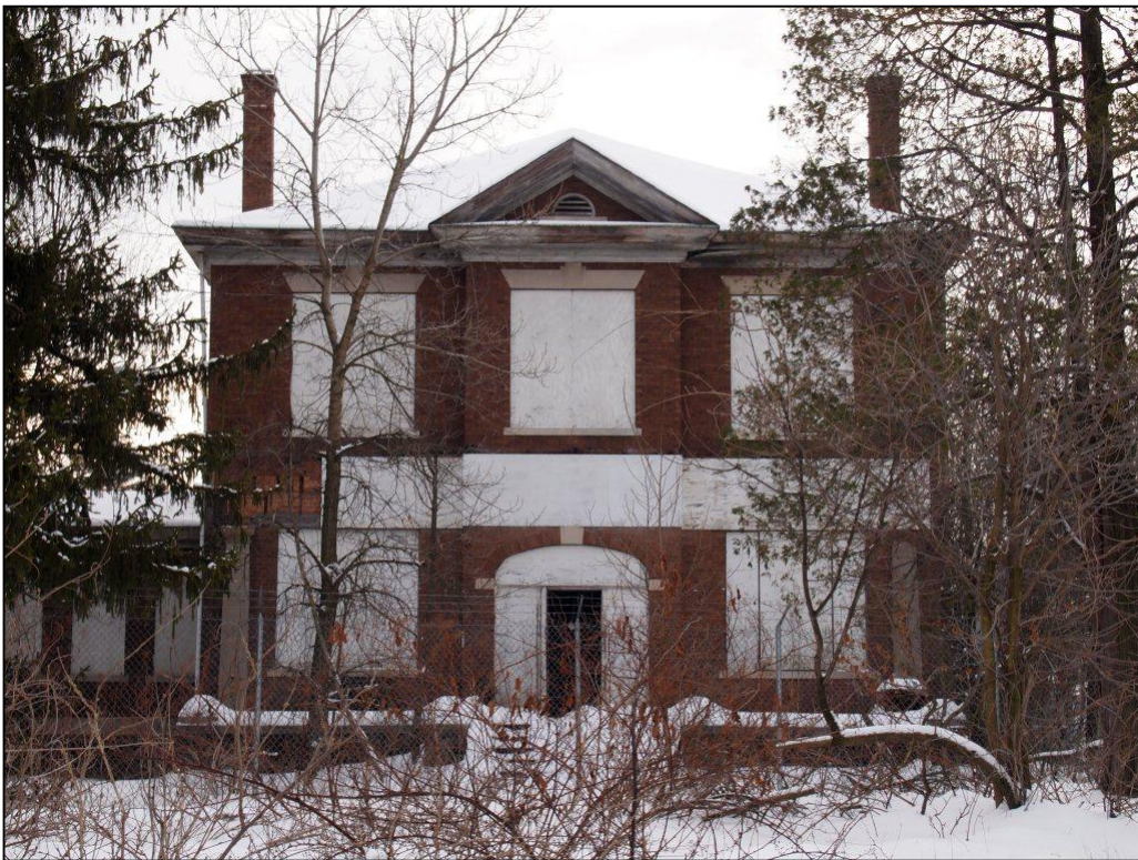
12. Beaver County Home. View southeast of front façade of west wing.
