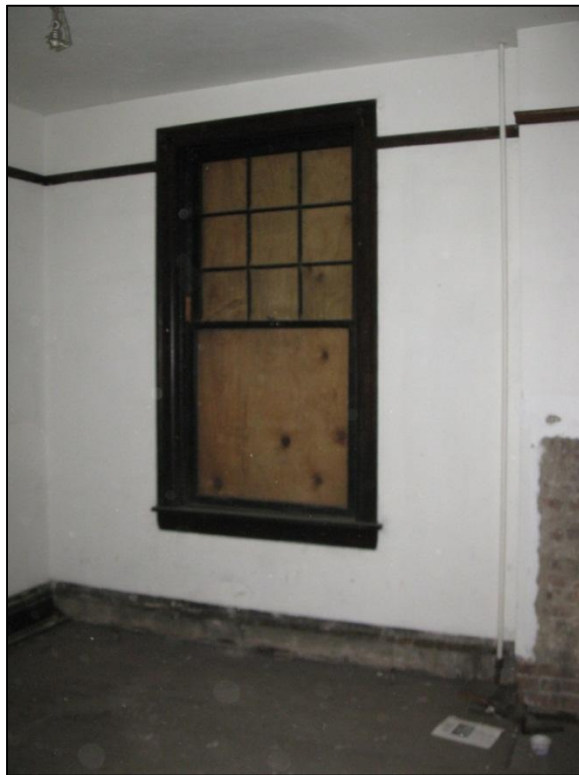
32. Beaver County Home. View of window in former dining room.
