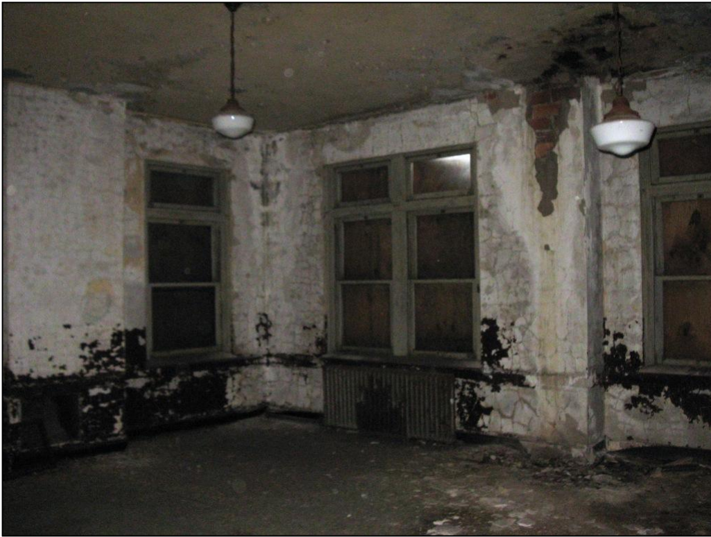
35. Beaver County Home. View of dormitory room in east wing.
