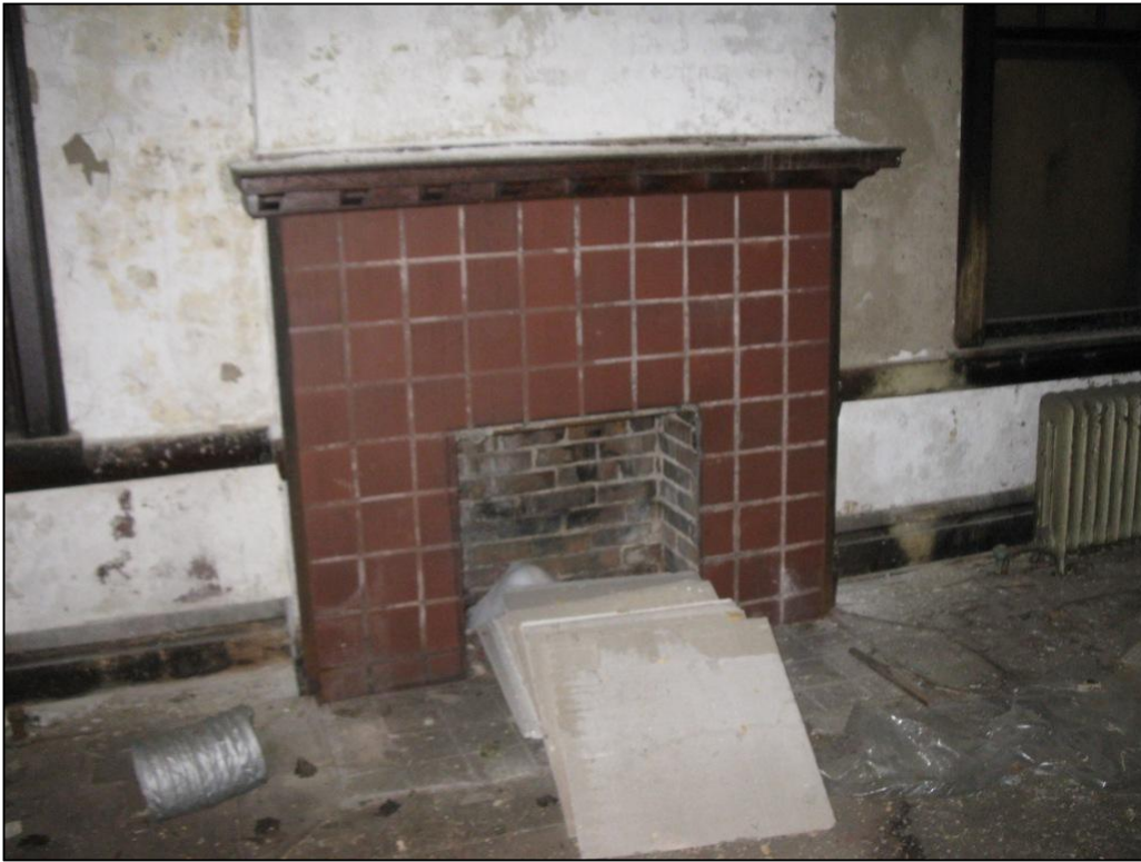
29. Beaver County Home. View of fireplace in former library.
