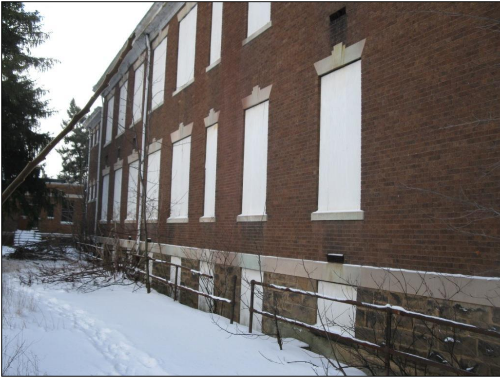
9. Beaver County Home. View southeast of side façade of east wing.
