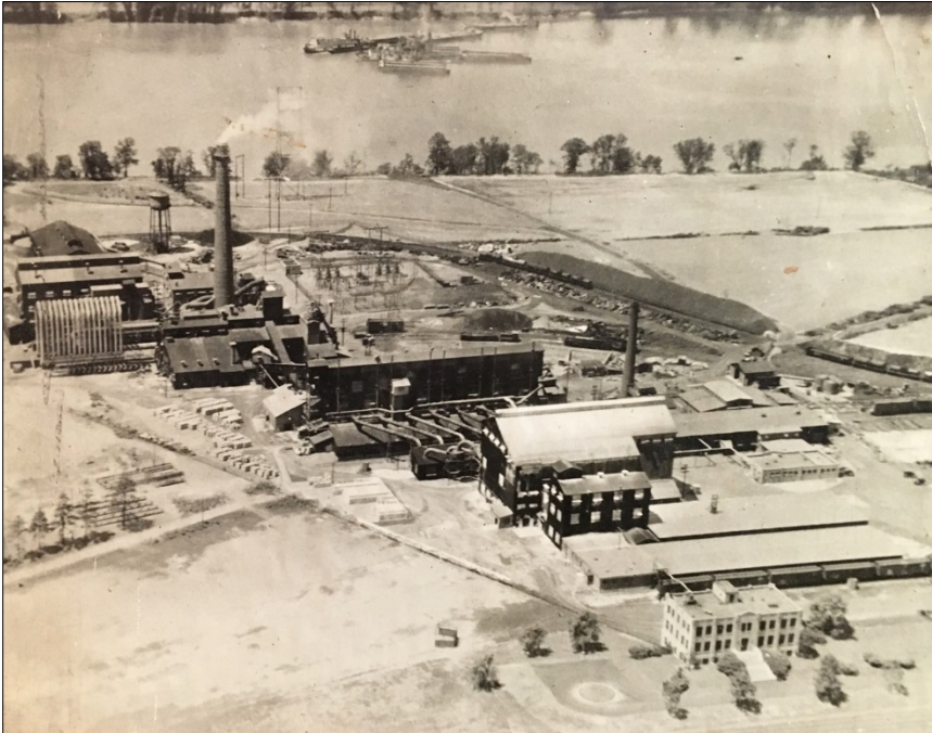
Figure 11. Aerial view of Josephtown Smelter, 1930s.
