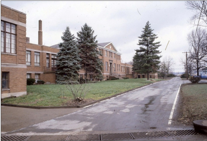
Figure 30. Main offices and laboratory space (former Beaver County Home and Hospital, which was acquired and partially renovated for use in 1964).
