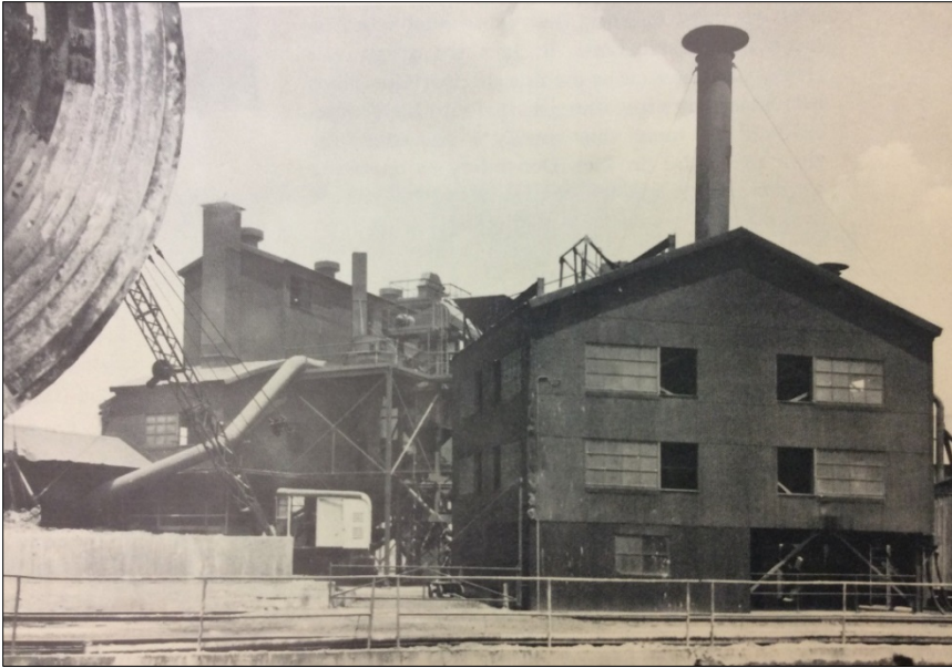
Figure 20. Secondary materials plant, 1955.
