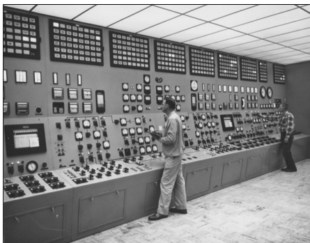
Figure 29. Power plant controls.
