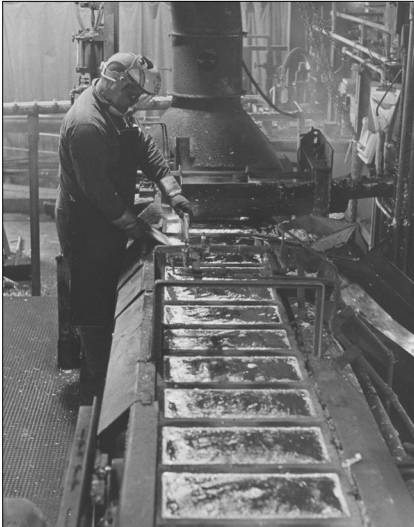
Figure 17. Casting zinc metal into slabs, c. 1964.
