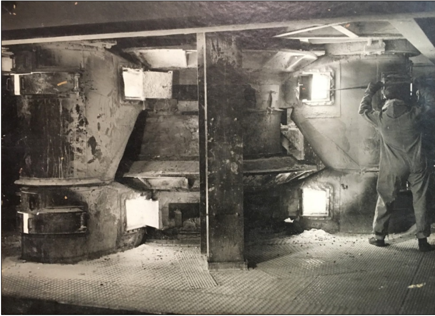
Figure 18. Blowing air into the oxide furnace with tuyeres, 1930s.
