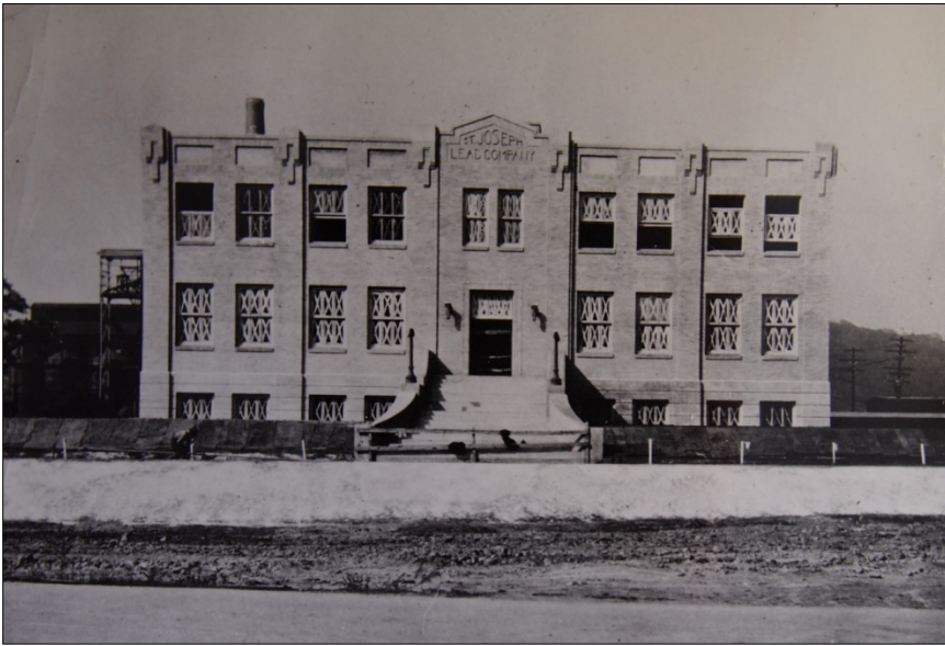
Figure 7. Office building nearing completion, October 15, 1930.
