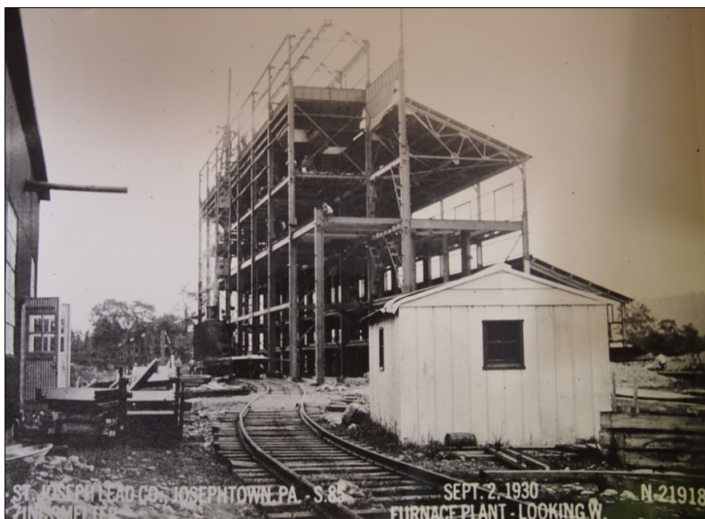
Figure 5. Furnace plant construction, September 2, 1930.
