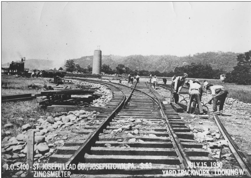
Figure 4. Yard track work and 300-foot stack under construction, July 15, 1930.
